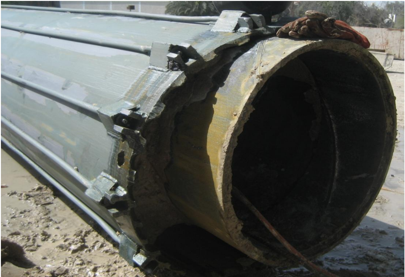
Figure 14. Extraction of the casing pile along with the existing pile.
