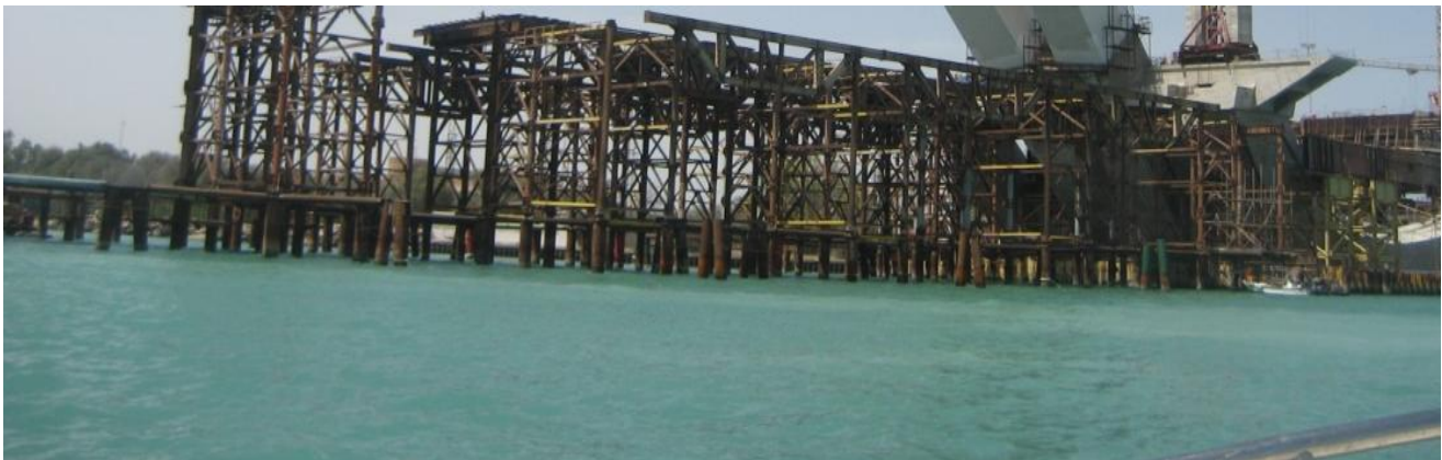
Figure 1. Temporary works – Falsework Erection on Piles.
