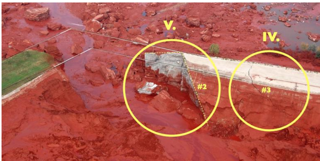
Figure 17. The fractures at Locations IV and V are hybrid fractures caused by the outflowing pressure of the red sludge and the additional settlement. These fractures occurred after the breach of the dam and they have no relevance to the failing of the dam. (Source: https://commons.wikimedia.org/wiki/File:Ajka_accident_d7df9fea08_b.jpg .)
