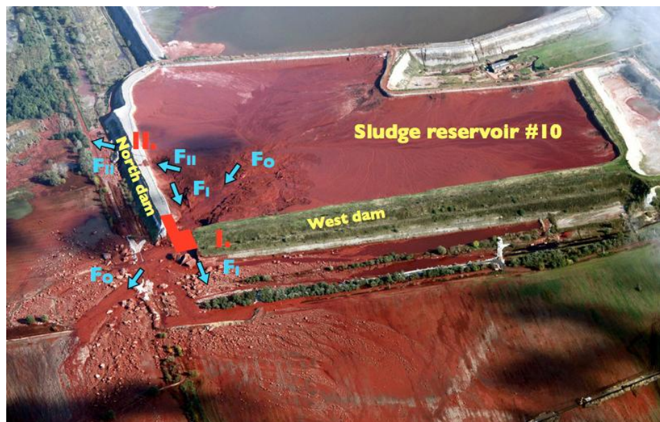
Figure 11. Based on the created flow channels in the red sludge, the flow directions were reconstructed. The initial flows F_1 and F_2 occurred at Locations I and II, pointing toward the direction of the existing fractures. The direction of flow F_1 changed to F_0 when the western part of the North dam had been washed away, creating a big opening. (Source: https://www.ndtv.com/world-news/hungarys-toxic-sludge-spill-as-big-as-gulf-oil-leak-435094 .)
