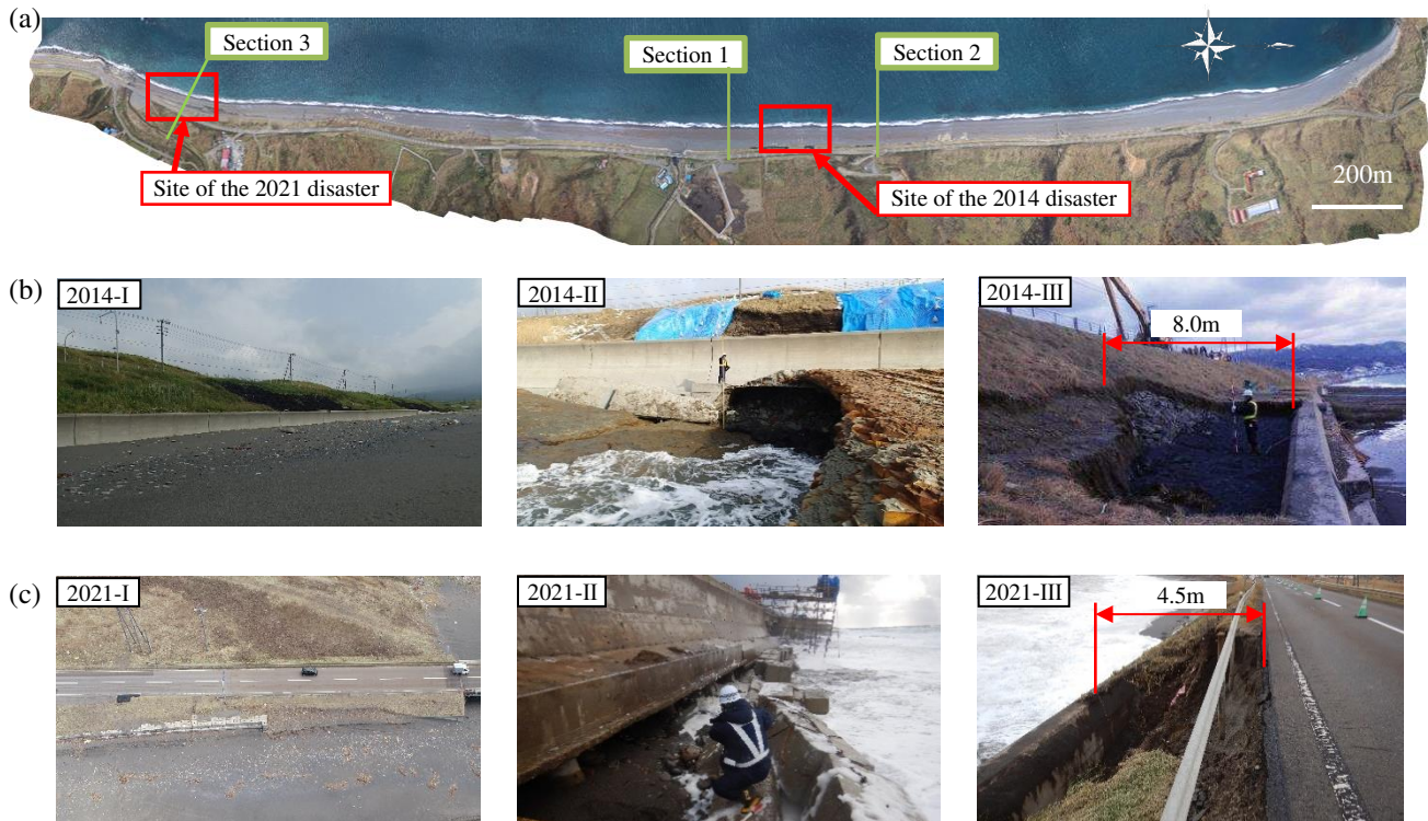
Figure 2. Field surveys of the 2014 and 2021 disasters: (a) Locations of foreshore slope surveys, (b) Situations at normal times (2014-I) and following the 2014 disaster (2014-II, 2014-III), and (c) Situations at normal times (2021-I) and following the 2021 disaster (2021-II, 2021-III).
