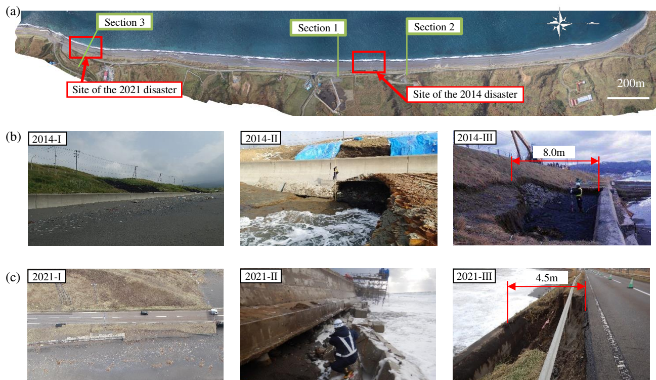
Figure 2. Field surveys of the 2014 and 2021 disasters: (a) Locations of foreshore slope surveys, (b) Situations at normal times (2014-I) and following the 2014 disaster (2014-II, 2014-III), and (c) Situations at normal times (2021-I) and following the 2021 disaster (2021-II, 2021-III).
