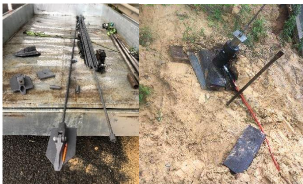
Figure 5. Percussion anchor (180-millimeter head) and load testing.
