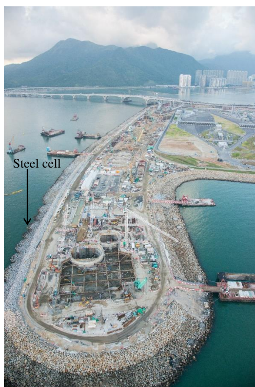
Figure 7. Southern Landfall reclamation in July 2018.
