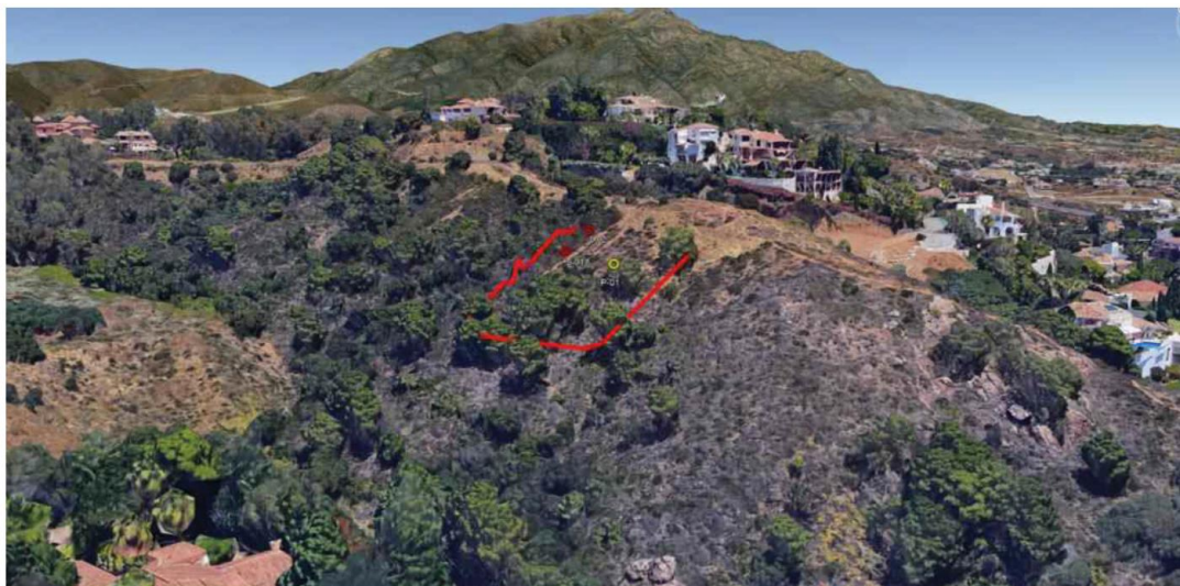
Figure 9. Northbound view of The Hills Plot 8 project.
