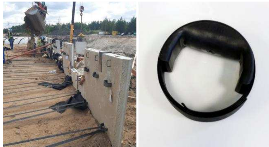
Figure 4. Geostrip reinforcements connected to the loop (on the right) and extending from rear of panel.
