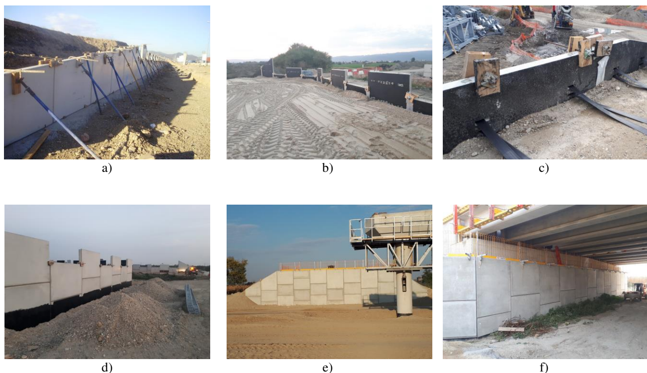
Figure 9. D4R7 Project VSoL® reinforced soil bridge abutment construction stages: (a) 1 st panel row installation, (b) backfilling, (c) polymeric strips placement, (d) frontal embedment detail, (e) frontal view, and (f) bridge deck arrangement.
