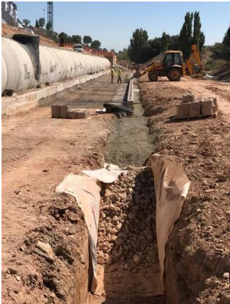
Figure 2. Different phases of the erection of Wall 1
