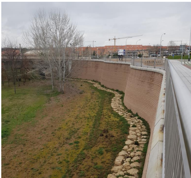
Figure 7. Wall 1 at the present time (Huesker geosintéticos).
