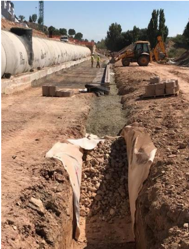
Figure 2. Different phases of the erection of Wall 1
