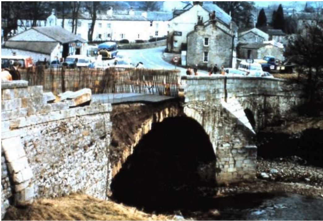
Figure 9. Failure of spandrel wall, Kettlewell New Bridge, 1984.
