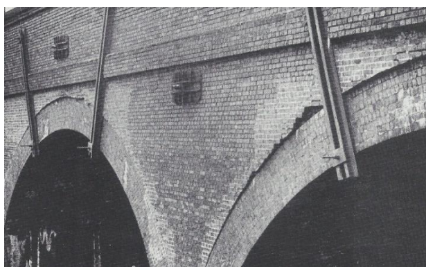
Figure 6. Tie-bars and spreader beams used to stabilize spandrel walls (Sowden and Jones, 1990).
