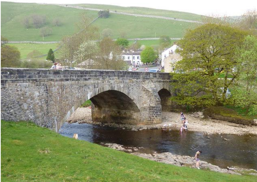
Figure 8. Kettlewell New Bridge, North Yorkshire, UK (Photo © Stephen Craven (cc-by-sa/2.0) ).
