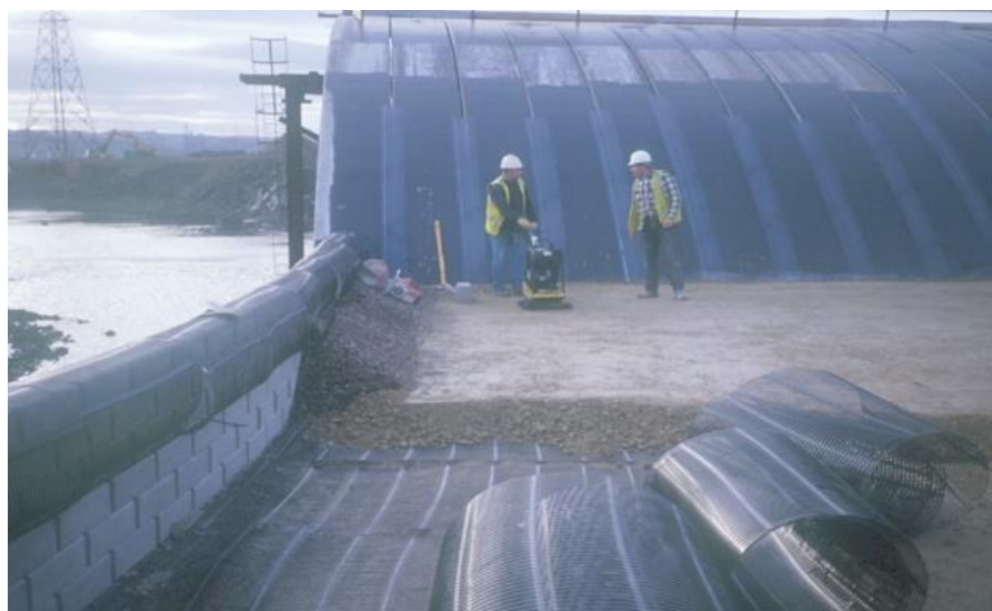
Figure 14. Construction of the soil reinforced masonry spandrel walls.
