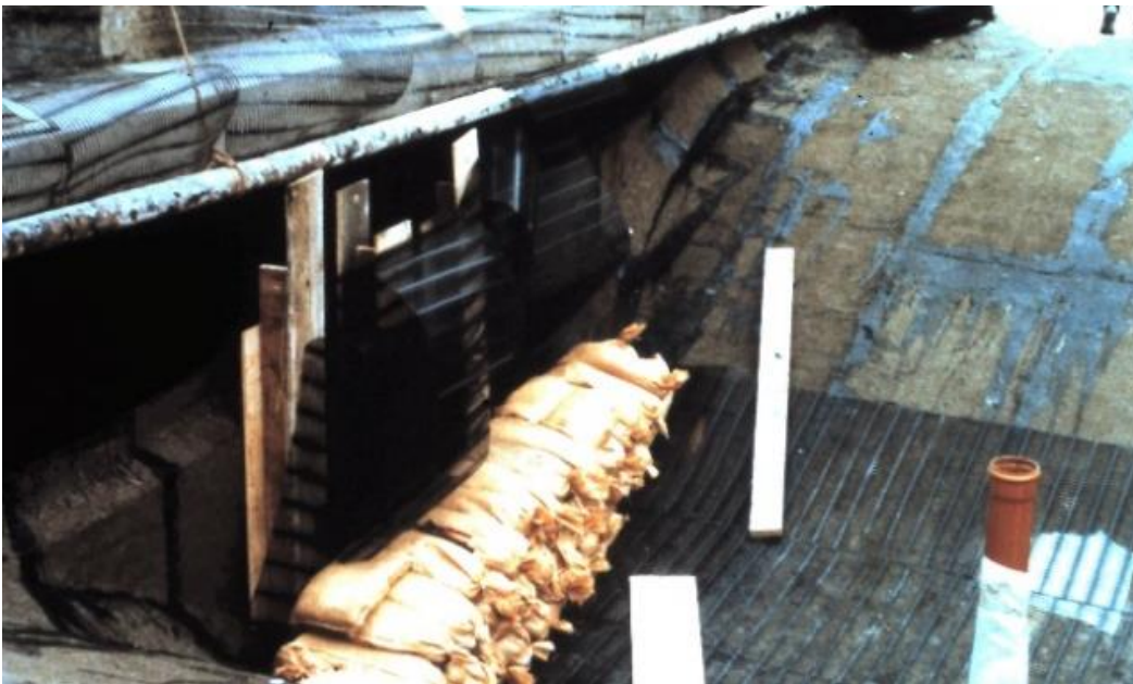
Figure 10. Construction of geogrid reinforced infill to spandrel walls, Kettlewell New Bridge, 1984.
