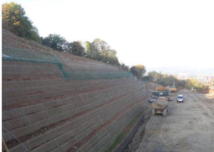
Figure 2. 17 m high structure constructed from draining geogrid and site won fill, Palmerston Park, Devon, October 2016.
