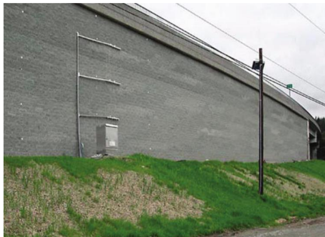
Figure 2. Photograph of 10.7 m-high MSE wall (Wall C) (Allen and Bathurst 2014a).
