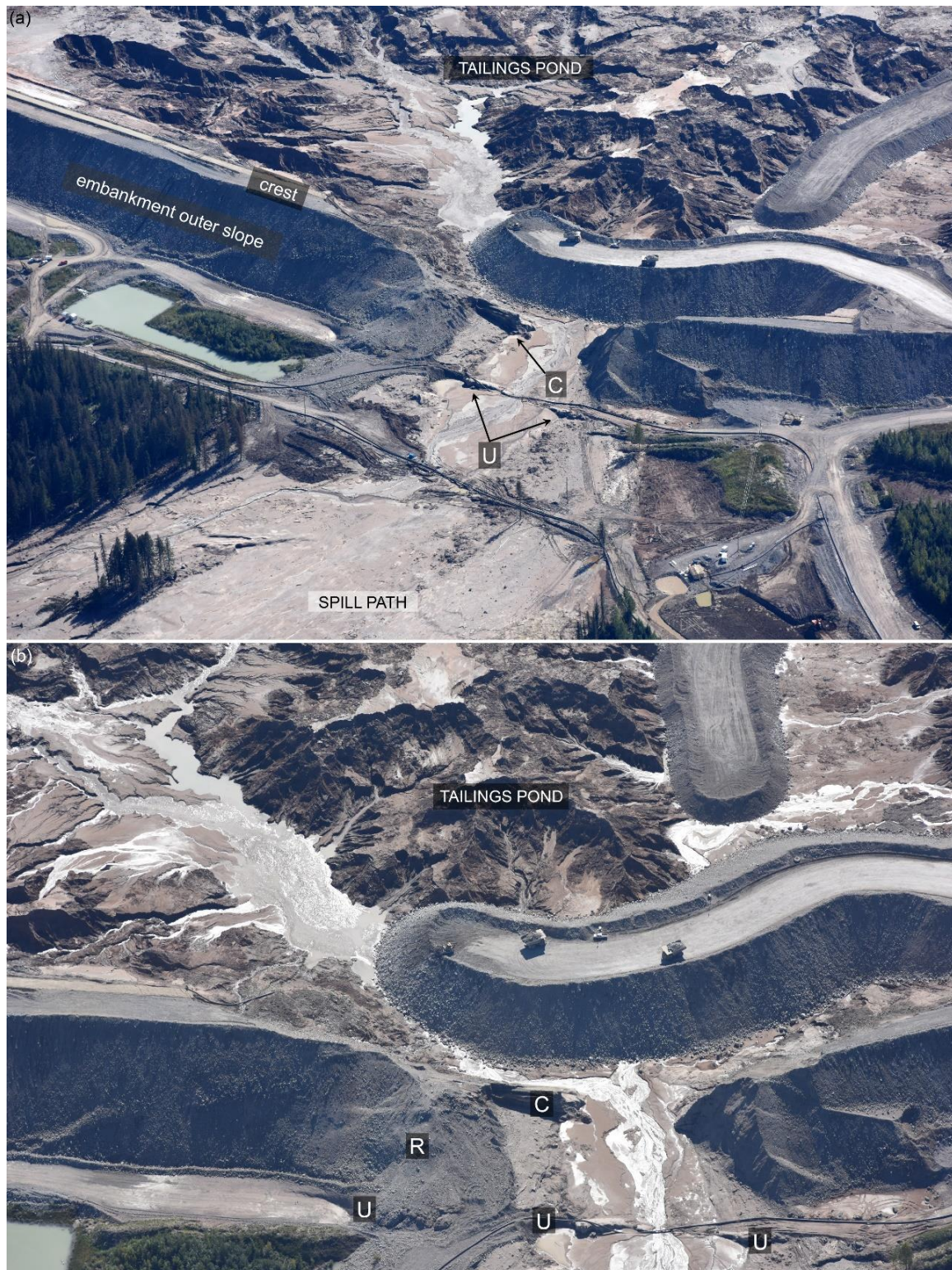
Figure 4. (a) Aerial diagonal view of the breach and spill path areas; (b) Aerial diagonal close-up of the breach location. Labels: C – core remnant, R – rockfill at the east boundary of the slide, U – uplift at the toe of the slide. Photography courtesy of Jamie Heath of terrasaurus.ca, taken 09/05/2014, reproduced with permission, altered to add labels.
