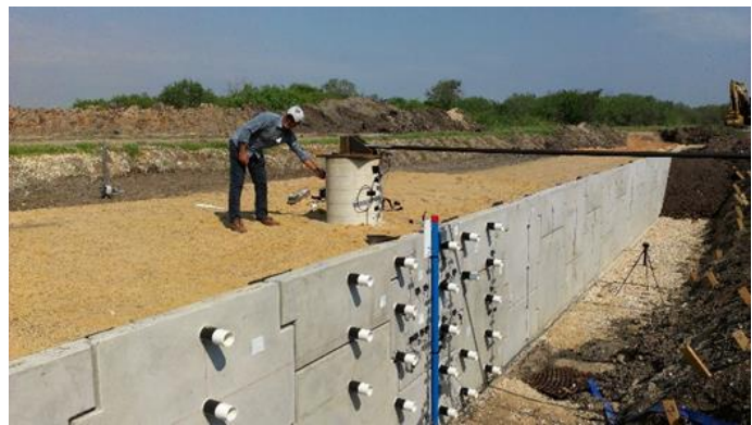
Figure 30. Construction of the MSE wall.
