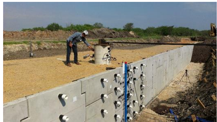
Figure 30. Construction of the MSE wall.
