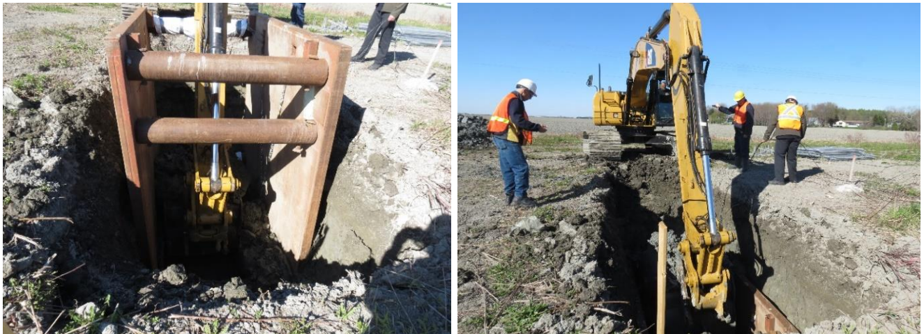
Figure 11. Excavation continued to make room to accommodate the second (upper) trench box in the trench.
