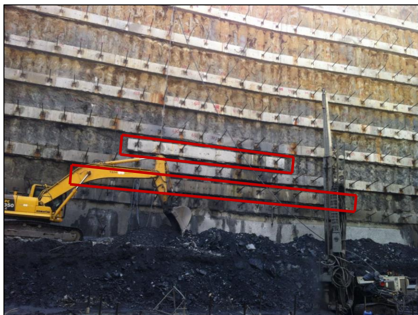
Figure 11. Additional Anchors on Section 3.
