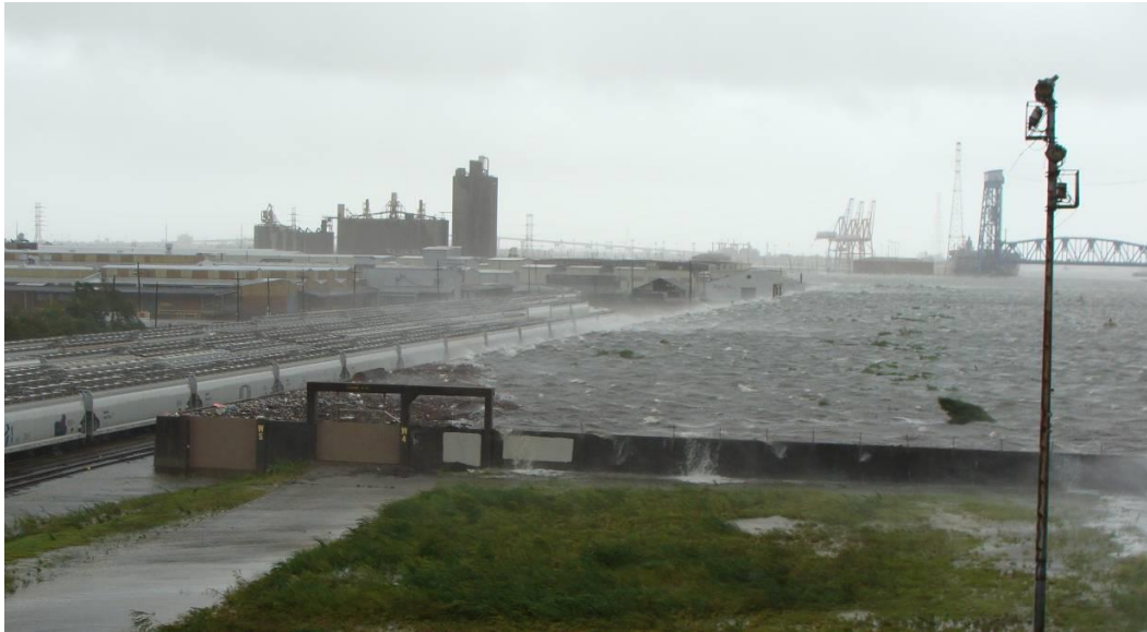
Figure 21. Photograph from September 1, 2008, of Gustav's storm surge. Photograph taken from Claiborne Ave. Bridge looking north. The waves are overtopping the T-wall. (September 1, 2008, 29.969° N, 90.027° W, USACE)
