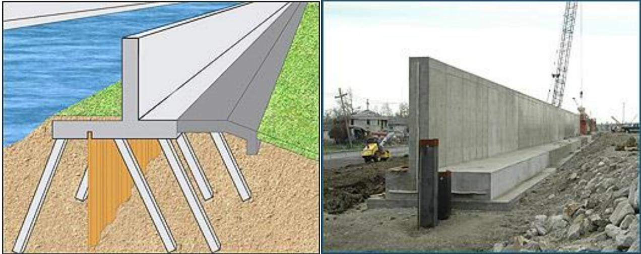
Figures 4 and 5. T-wall schematic and photograph of T-wall under construction.
