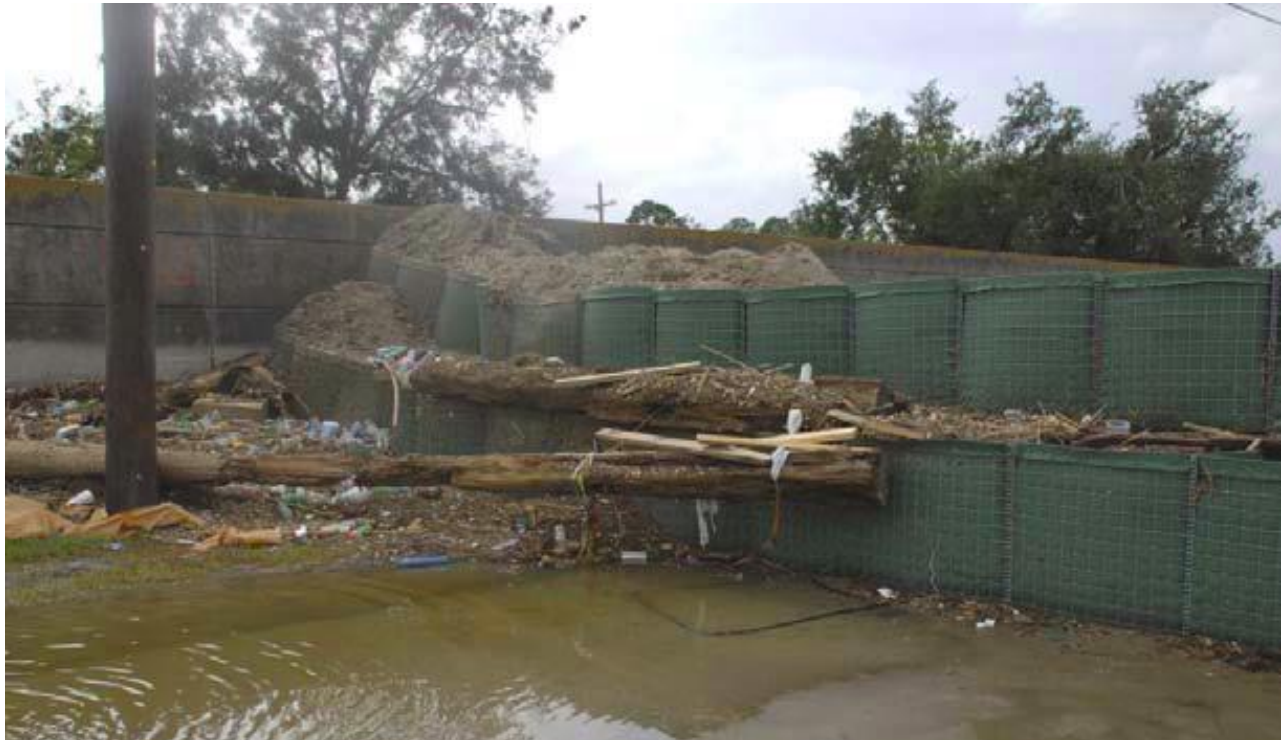
Figure 31. End of temporary bin wall at tie-in to I-Wall, post-Gustav (September 2008, 30.0122° N, 90.0313° W, http://www.mvn.usace.army.mil/HPS/Status%20Report%20Newsletters/Sept_9_2008.pdf )
