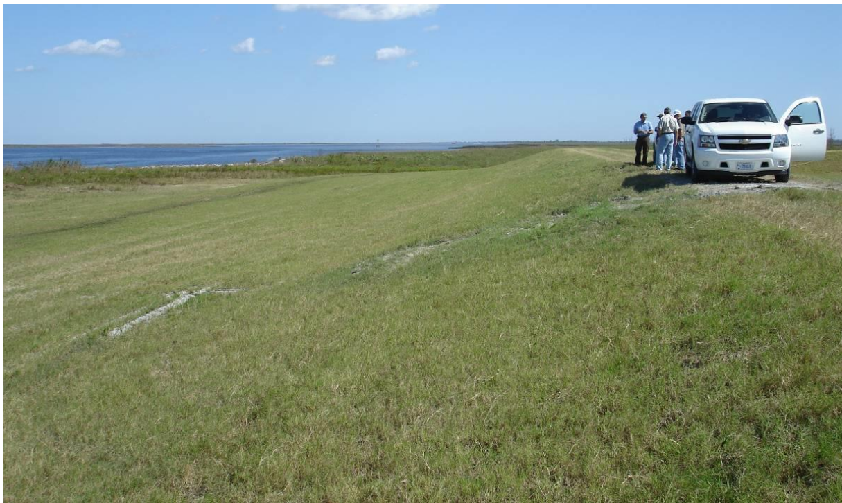
Figure 3. Southeast corner of the MRGO levee, flood side. (October 2, 2008, 29.8889°N, 89.7617°W)
