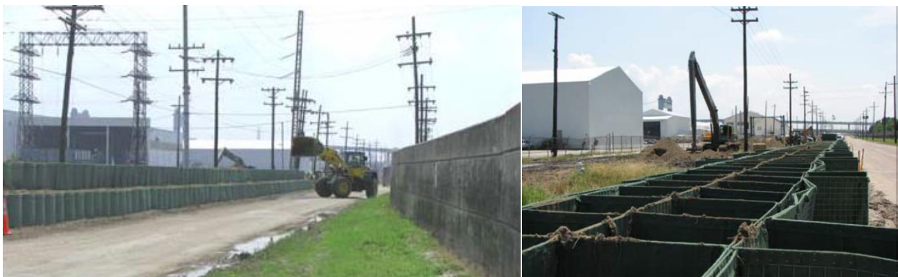
Figure 30. Temporary bin wall under construction, IHNC West along France Road. (August 2008, 30.0157° N, 90.0324° W, http://www.mvn.usace.army.mil/HPS/Status%20Report%20Newsletters/Sept_9_2008.pdf )
