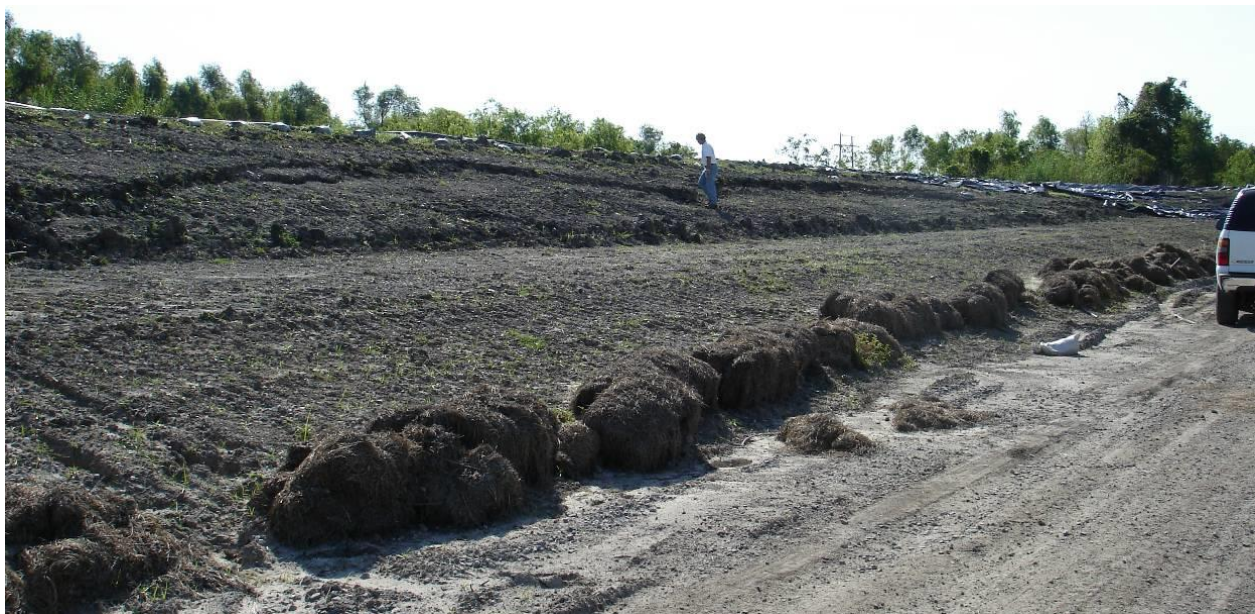
Figure 35. Protected side slope of the Plaquemines Parish back levee and slide. (October 3, 2008, 29.8506° N, 89.9085° W)
