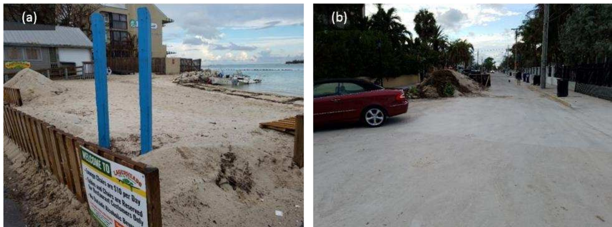
Figure 10. (a) Simonton Beach was severely eroded and (b) sediment was deposited in the parking lot backing the beach (collected September 27, 2017; location 24^{\circ}33'42.85''N , 81^{\circ}48'19.64''W ).
