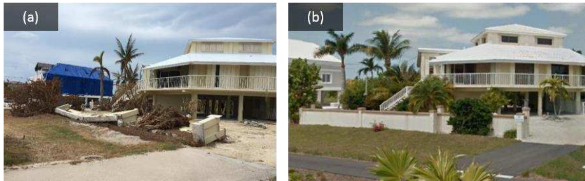
Figure 14. (a) A wall located in front of a home on Sombrero Beach Road collapsed during Hurricane Irma (collected September 26, 2017; location 24^{\circ}41'34.26''N , 81^{\circ}5'0.93''W ); (b) the pre-existing structure appeared to be intact prior to the storm. Map Data: Google (2018).
