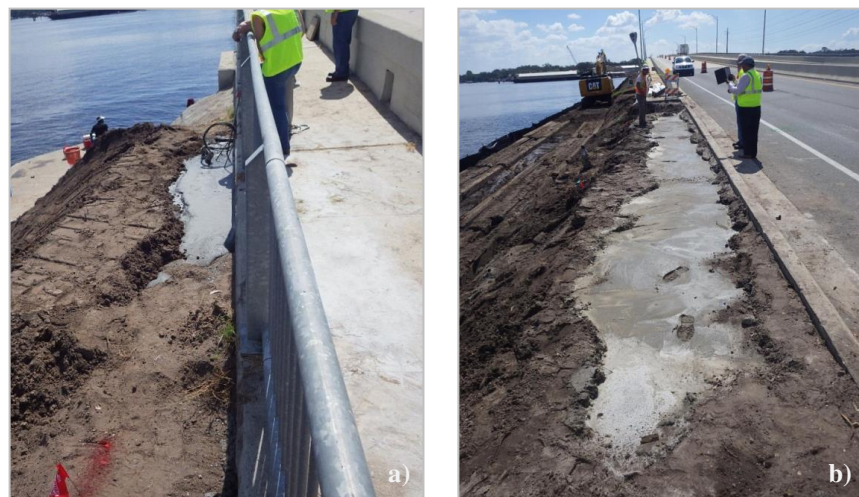
Figure 23: Repaired northeastern bridge embankment for US 17 bridge over the Trout River at 30^{\circ}23'45.44''\text{N} latitude and 81^{\circ}38'53.95''\text{W} longitude that includes the rebuilt soil and excavatable flowable fill trench embankment (a) adjacent to the concrete covered, stacked concrete sack wall; and (b) roadway edge (Hudyma et al., 2017).
