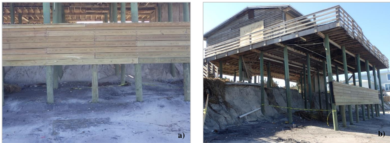
Figure 11. (a) Shallowly embedded timber seawall at approximately 29°56'49.30"N latitude and 81°18'9.37"W longitude, showing significant erosion (about 2 m or 6.6 ft) below a residential structure; and (b) subsequent beach erosion and removal of the first story walls by wind and water.
