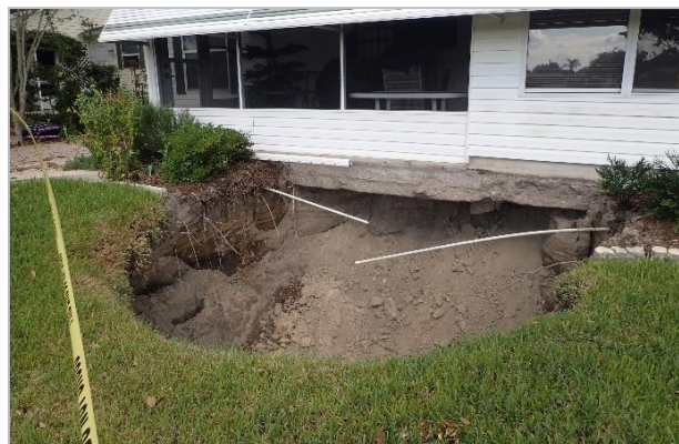
Figure 6. Sinkhole undercutting a foundation at 2536 Botello Road at 28°57'11.67"N latitude and 81°59'30.05"W longitude (Hudyma et al., 2017).
