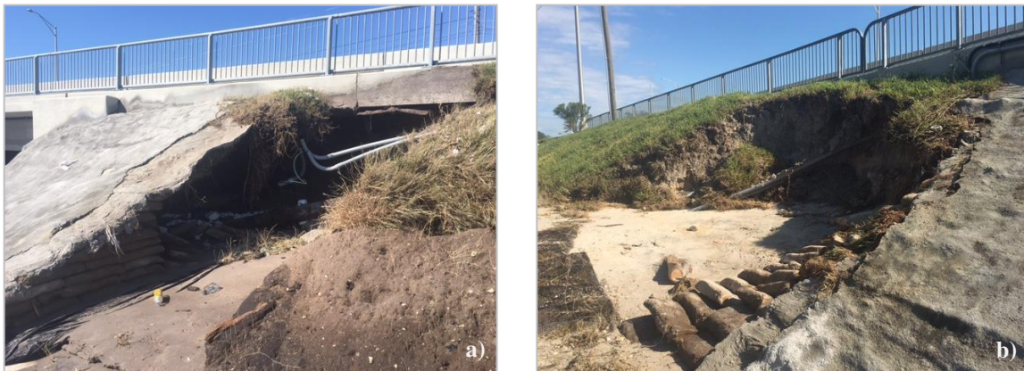
Figure 22. Scour damage along the (a) northeastern and (b) northwestern bridge embankment of the US 17 bridge over the Trout River at 30^{\circ}23'44.43''\text{N} latitude and 81^{\circ}38'54.13''\text{W} longitude (Hudyma et al., 2017).
