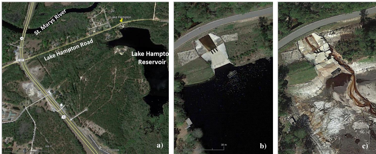
Figure 14. (a) Lake Hampton Dam reconnaissance site location with aerial photos of the dam (b) before (March 2017), and (c) after (October 2017) the failure (Google Earth 2018).
