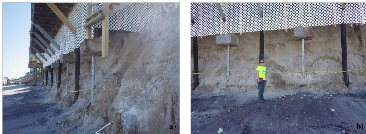
Figure 10: Erosion undercutting both the timber pile supports and micropile supported concrete footings for a beach house with continued slope failures in drying sand at 29^{\circ}56'47.00''\text{N} latitude and 81^{\circ}18'8.10''\text{W} longitude after Hurricane Irma.
