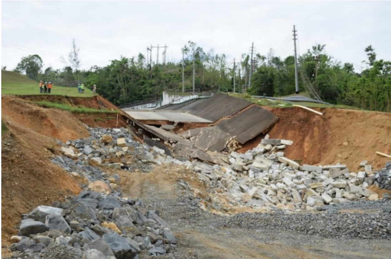
Figure 10. Damaged condition of Guajataca Dam spillway (Silva-Tulla et al., 2018).
