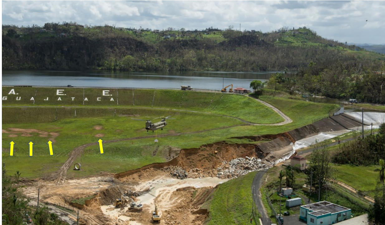
Note: Yellow arrows show location of apparent sand boils downstream of the dam toe.
