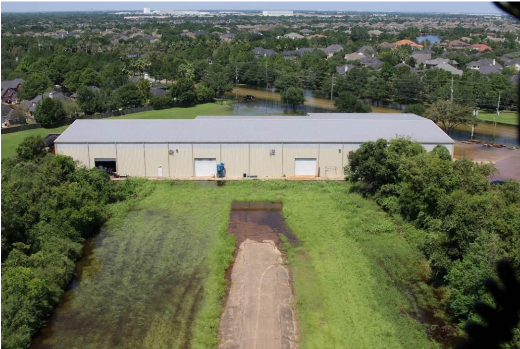
Figure 8. North end of Addicks auxiliary spillway (September 3, 2017, 29.84977° N, 95.58904° W, photo by USACE).
