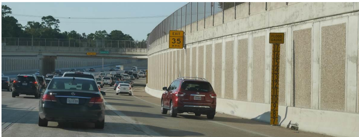
Figure 31. Beltway 8 / Boheme Drive underpass and flood depth signs (September 11, 2017, 29.76694° N, 95.56139° W).
