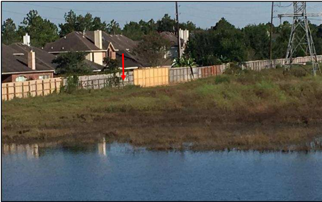
Figure 11. High water mark on fences surrounding residential area (September 9, 2017, 29.70706° N, 95.72835° W).
