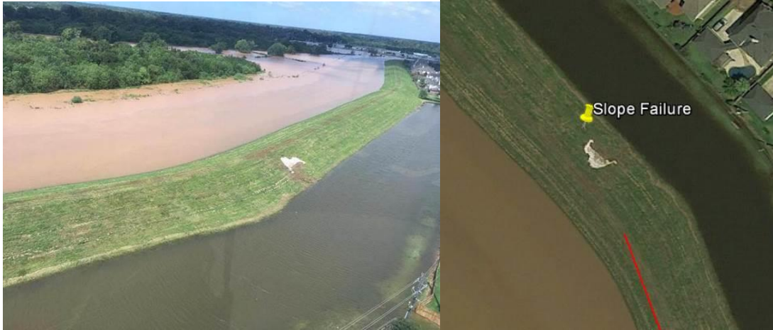
Figure 14. Aerial photo (right) and Google Earth (left), August 30, 2017, 29.491844° N, 95.541017° W.
