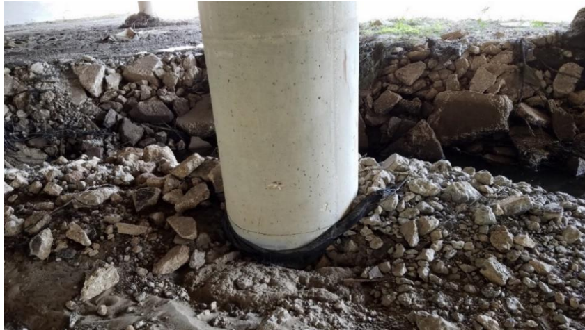
Figure 38. Erosion control riprap, including polymeric reinforcement, with minimal observed scour (September 11, 2017, Time 10:19 CDT, 30.24688° N, 95.45796° W).
