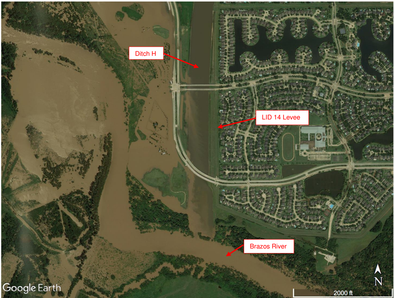
Figure 17. A Google Earth image of LID # 14 and Ditch H and its connection to the Brazos River (August 30, 2017).
