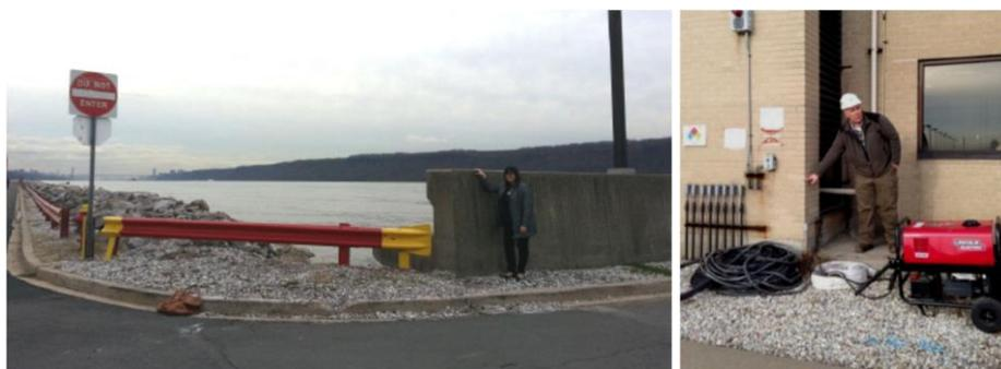
Figure 27. Yonkers Joint WWTP: junction of rip-rap revetment and seawall, looking south (left); vent grates in aeration blower building where water entered, with flood water elevation shown by plant superintendent (right); GEER (2014).
