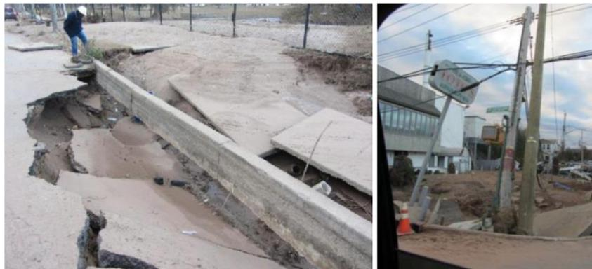
Figure 24. Scour undermining of street and utilities at Seaview Blvd, SI (40.579283°N, 74.077849°W, 11/4/12, GEER, 2014).
