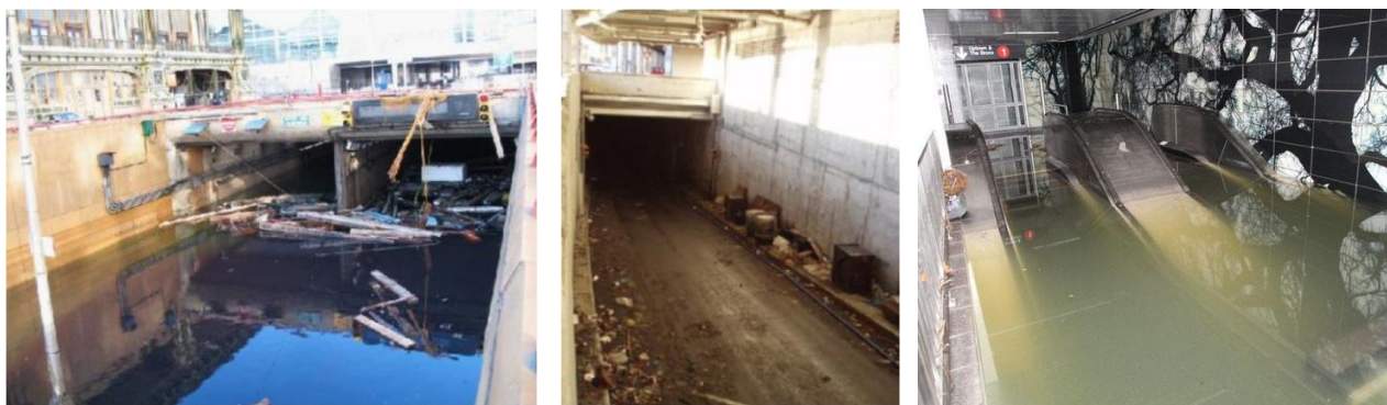
Figure 13. Flooded Battery Park underpass (40.701600°N, 74.011742°W) on 11/4/12 (left, by GEER 11/3/12); E30 th St. (40.739830°N, 73.973263°W) Bellevue Hospital (middle, by GEER 11/3/12); South Ferry station (right, by MTA 10/30/12).
