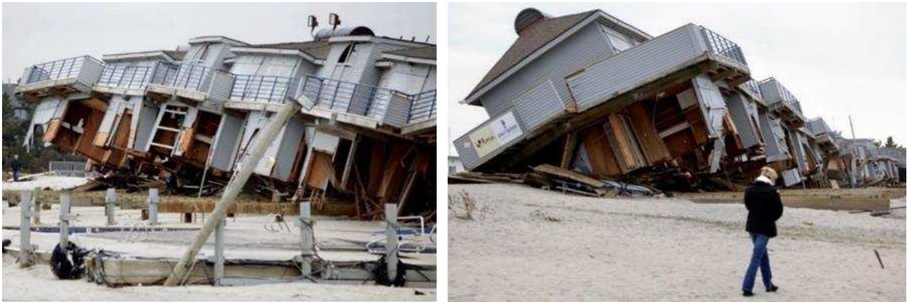
Figure 19. Sea Bright, NJ, beach cabana (40.350086°N, 73.972954°W) pulled off its base (Photo by AP/Wenig; 11/19/12).
