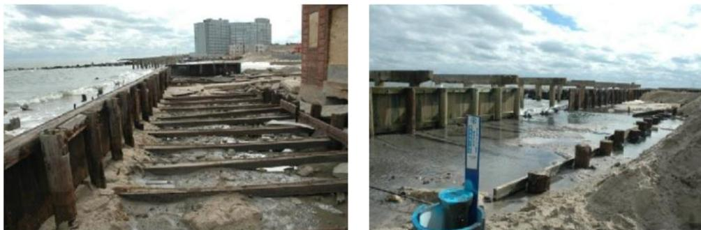
Figure 25. Bulkhead in Atlantic City, NJ: backfill soil washed away, exposing severely corroded tie rods (GEER, 2014).
