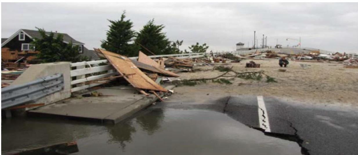
Figure 10. Foundation undermining at east abutment of Mantoloking Bridge ( $40.040058^{\circ}\text{N}$ ,  $74.051886^{\circ}\text{W}$ ; GEER, 2014).
