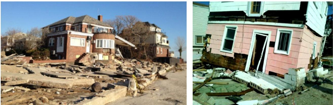
Figure 20. Undermining of beachfront retaining wall and loss of retained soil, Sea Gate, Brooklyn (left, 11/9/12); Destroyed CMU wall foundation, Breezy Point, Queens (right, 11/12/12). Photos by NYCDob (GEER, 2014).
