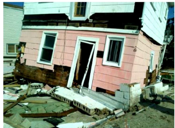
Figure 20. Undermining of beachfront retaining wall and loss of retained soil, Sea Gate, Brooklyn (left, 11/9/12); Destroyed CMU wall foundation, Breezy Point, Queens (right, 11/12/12). Photos by NYCDob (GEER, 2014).
