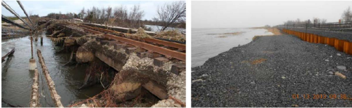
Figure 16. Earth embankment washouts in Queens, along Rockaway subway [A] line after Sandy with old LIRR infrastructure exposed (left) and post mitigation work (right). Photos by Khinda, ed. (2013).
