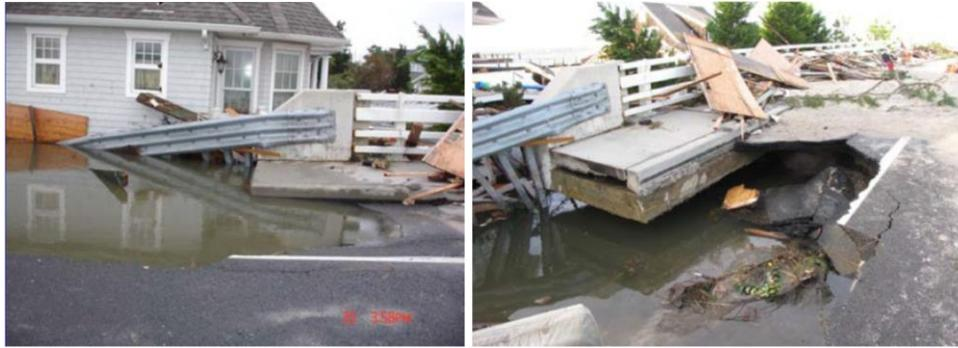
Figure 11. Mantoloking Bridge east abutment erosion (40.040058°N, 74.051886°W, Ocean Ct. Eng., 2012; GEER, 2014).
