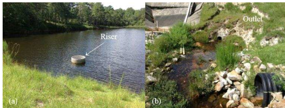
Figure 27. Primary spillway in Dam D: a) riser structure (southwest view from crest); and b) outlet pipe (southwest view from downstream).
