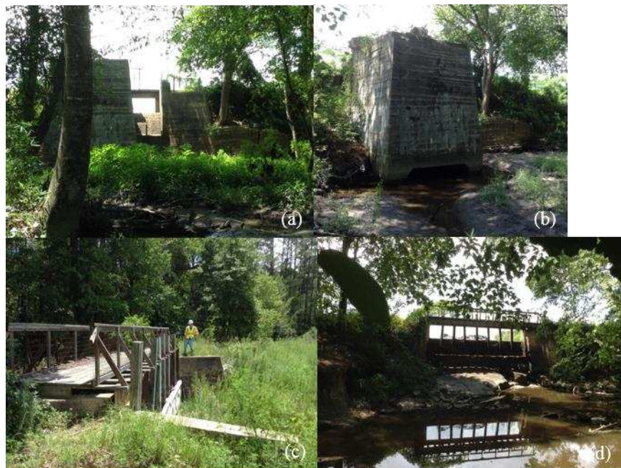
Figure 20. Spillways in Dam C: (a) first spillway structure (southwest view from downstream), (b) close up of concrete gate in first spillway structure (southwest view from downstream), (c) second spillway structure near the southeast end of the dam (southeast view from crest), and (d) southeast view of second spillway structure from downstream.
