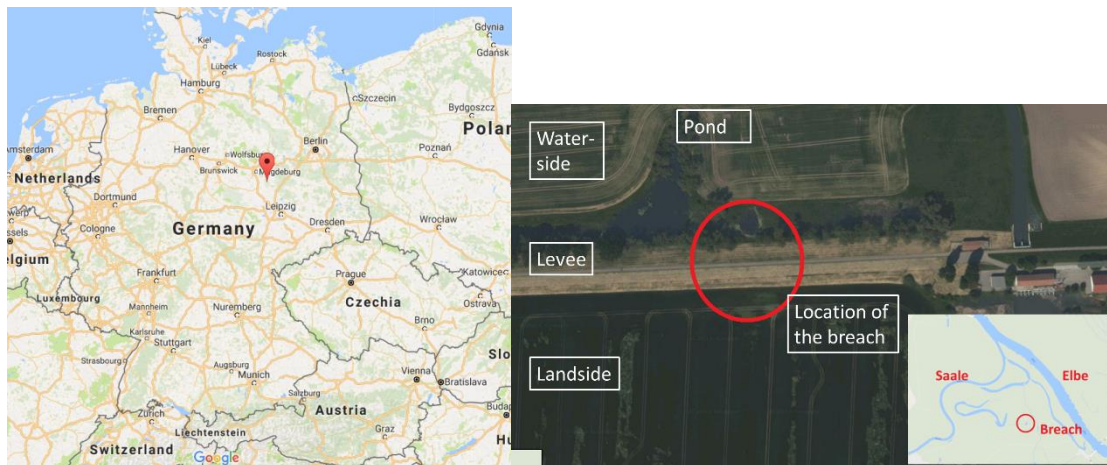
Figure 2. Overview of the location of the breach (GeoBasis-DE/BKG, 2009).
