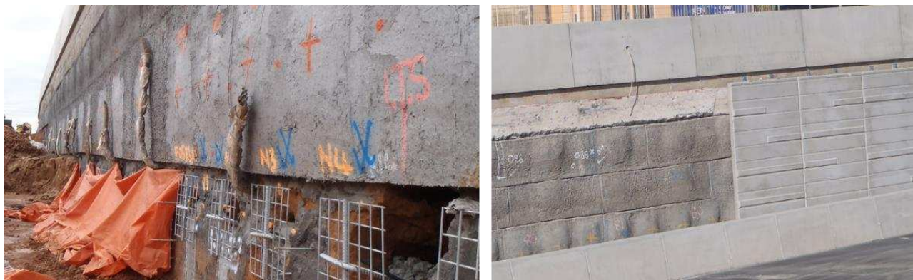
Figure 11. Photographs of wall prepared for shotcreting (left) and shotcreting completed with some facing panels installed (right).
