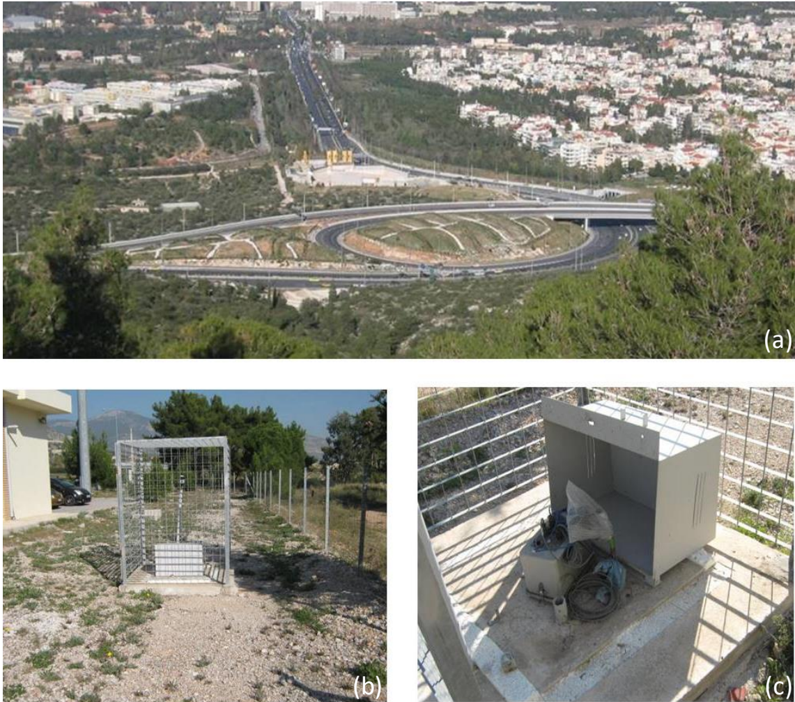
Figure 17. View of one accelerograph station. (a) The highway section monitored; (b) The station with the GPS antenna; (c) Close-up of Recording Instruments and wiring.
