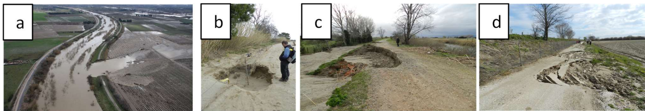
Figure 14. a) The March 2013 breach at the Pia location on the right of the river (photo: DREAL Languedoc-Roussillon), b) A sinkhole close to the breach (photo: Patrice Mériaux, Irstea), c) Damage caused by overflowing (photo: Patrice Mériaux, Irstea), d) Damage to a track on the landward side of the dike caused by under-seepage (photo: Patrice Mériaux, Irstea)
