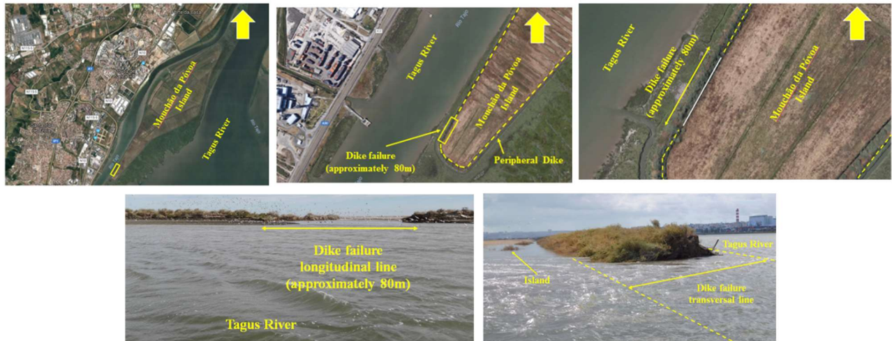
Figure 38. Location and view of the dike failure.
