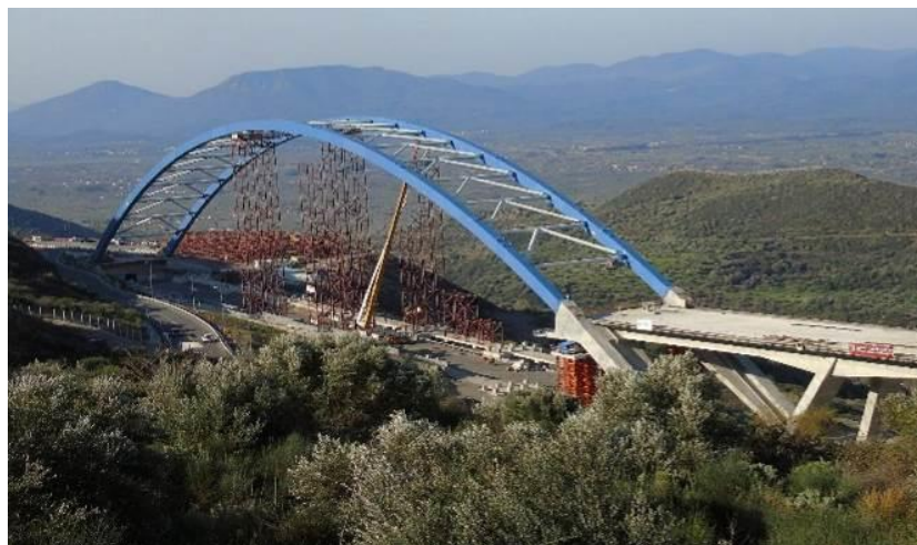
Figure 14. Removal of the temporary towers.
