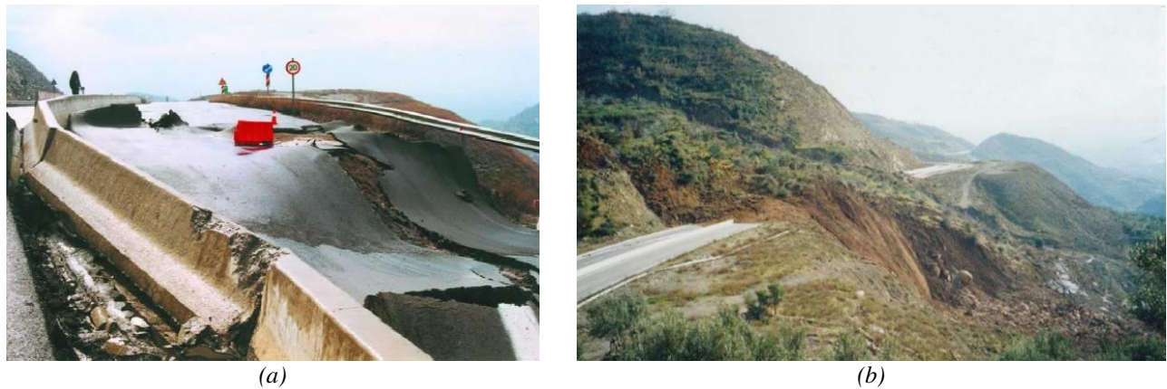
Figure 1. The Tsakona landslide (February 2003) (EMEK S.A (2015)) (a) large settlements on the road pavement (b) massive soil movement (Fikiris et al. (2001)).
