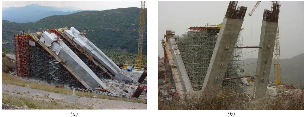
Figure 9. Construction of the (a) curved struts and (b) straight struts of the bridge pier.
