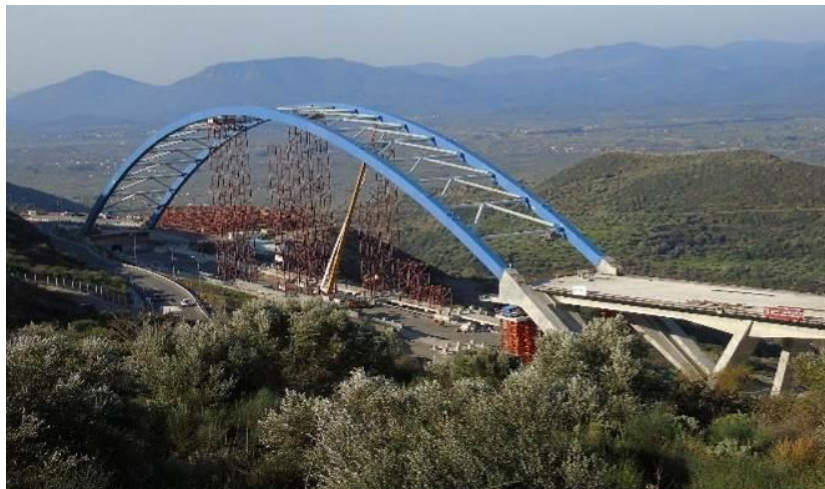
Figure 14. Removal of the temporary towers.
