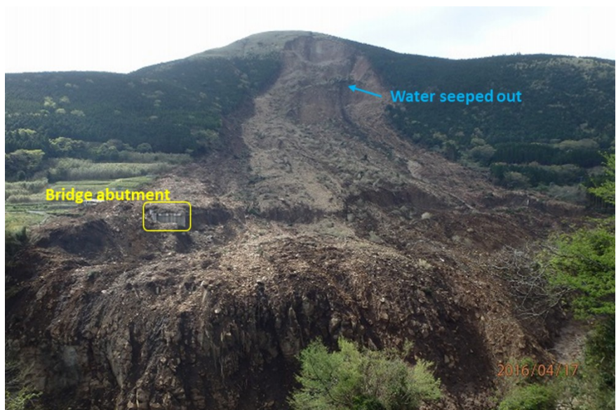
Figure 28. Landslide near Aso Ohashi Bridge (site 17 in Fig. 26). (32° 53'0.02"N, 130° 59'22.80"E).
