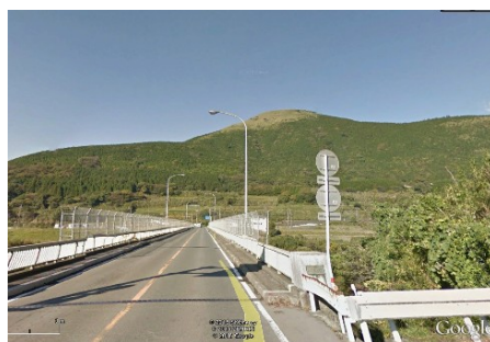
Before the failure (Google Earth)
