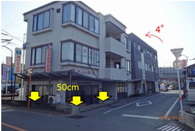
Figure 4. Liquefaction-induced damage to buildings in Karikusa district (Site 1 in Fig. 3) ( 32^{\circ} 45'35.70''N , 130^{\circ} 40'59.76''E ).
