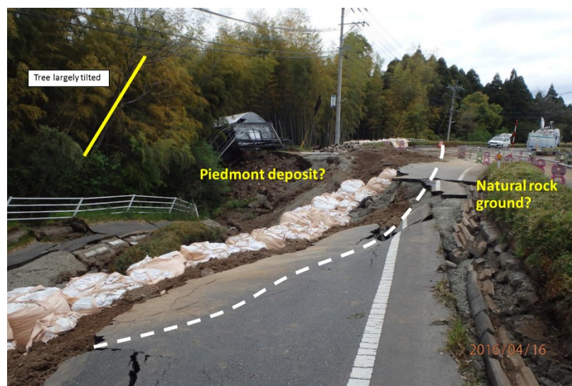
Figure 18. Damage to Route 443 in Mashiki Town (Site 10 in Figs. 12 and 14) ( 32^{\circ} 47'29.71''N , 130^{\circ} 49'17.58''E ).
