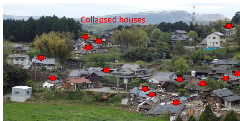
Figure 23. Damage to residential houses in Ohkiri-hata area (site 15 in Fig. 12) ( 32^{\circ}50'36.91''N , 130^{\circ}55'43.16''E ).
