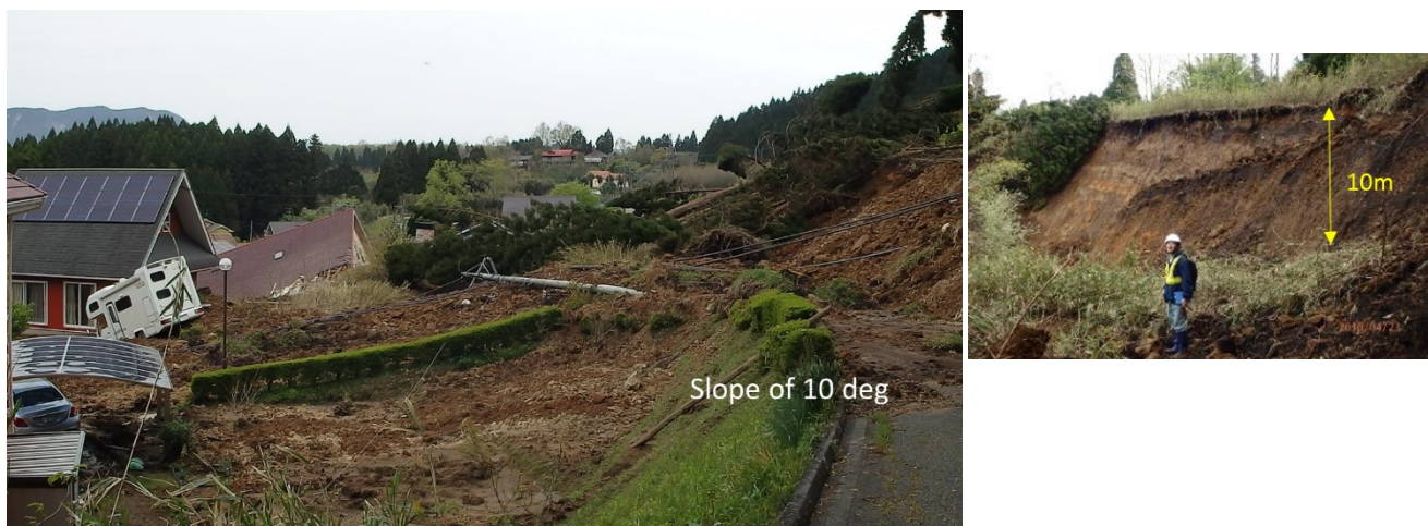
Figure 30. Landslide at gentle slope and its scrap (site 19 in Fig. 26) ( 32^{\circ} 52'29.42''N , 131^{\circ} 00'49.36''E ).
