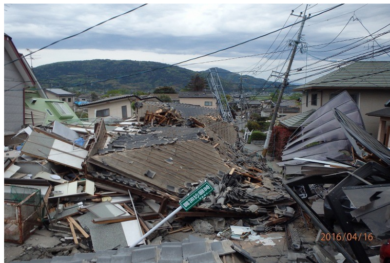
Figure 13. Damage to residential houses in Mashiki Town (Site 7 in Fig. 12) ( 32^{\circ} 47'16.38''N , 130^{\circ} 48'58.47''E ).
