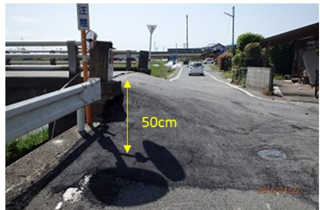
Figure 9. Temporary restoration work (filled slope) for settlement of levee (Site 5 in Figs. 3 and 7) ( 32^{\circ} 46'44.47''N , 130^{\circ} 47'45.43''E ).
