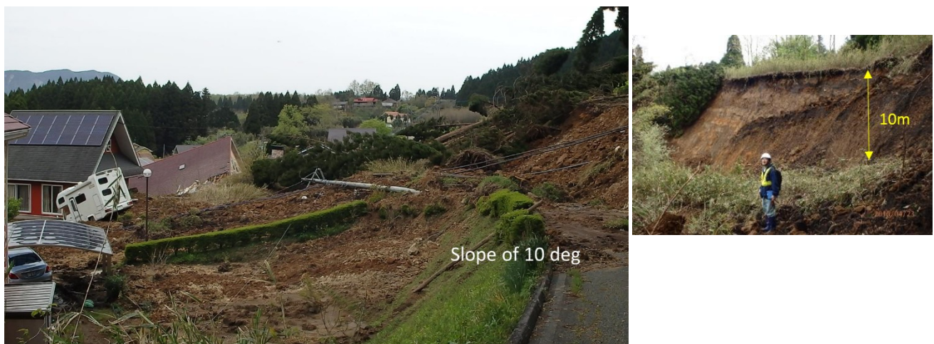
Figure 30. Landslide at gentle slope and its scrap (site 19 in Fig. 26) ( 32^{\circ} 52'29.42''N , 131^{\circ} 00'49.36''E ).
