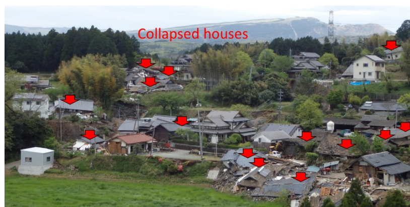
Figure 23. Damage to residential houses in Ohkiri-hata area (site 15 in Fig. 12) ( 32^{\circ}50'36.91''N , 130^{\circ}55'43.16''E ).
