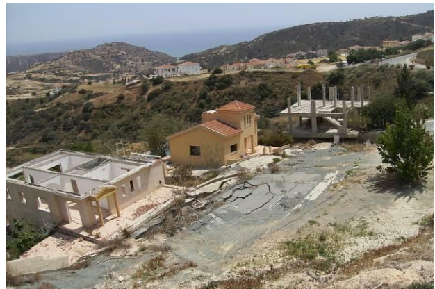
Figure 2. Left: Northward view of the Pissouri landslide. Dashed line marks the border of the sliding mass. Back scarp is also marked. Right: The distorted road and damaged buildings resting at the upper part of the sliding mass.
