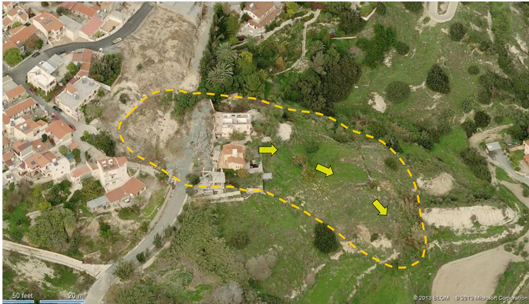
Figure 1. Aerial view of the Pissouri landslide. Dashed line indicates the border of the sliding mass. Notice the distorted road and the damaged residential buildings resting on the sliding mass.
