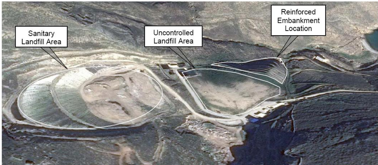
Figure 4b. Close up view of project location.
