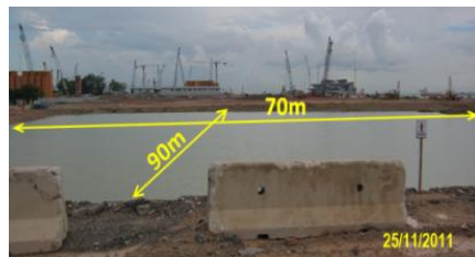
(a) Photograph of pond A (90 m x 70 m x 5.5 m) with slurry clay heaved from RL94.5 m to RL100 m.
