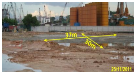
(c) Photograph of pond C. (37 m x 30 m x 7.5 m) with slurry clay heaved from RL94.5 m to RL102 m.
