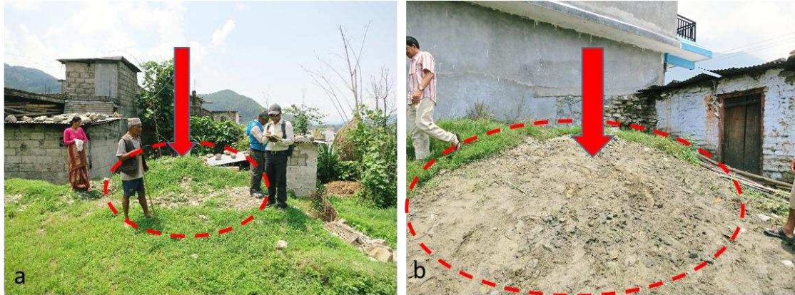
Figure 6. Typical effects of sinkhole formation on residential properties observed on June 2014 included the collapsed of (a) a cowshed and (b) a masonry kitchen.
