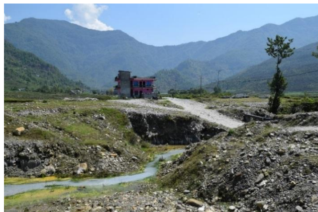
Figure 9. Muddy silty water observed in the sinkhole damaged area (photo point 7) following the 2015 Gorkha Nepal Earthquake.
