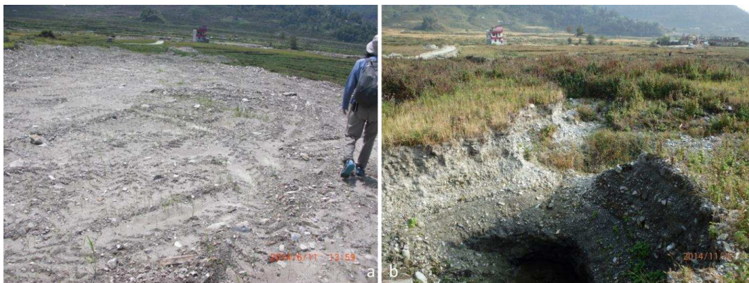
Figure 7. (a) Sinkholes backfilled area (photo point 5) as seen in June 2014; and (b) Re-activated sinkholes as observed in November 2014.
