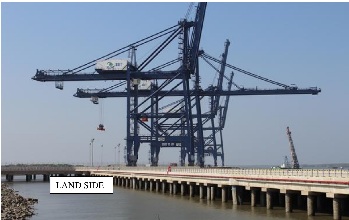
Figure 2. Photo of the berth area prior to use.
