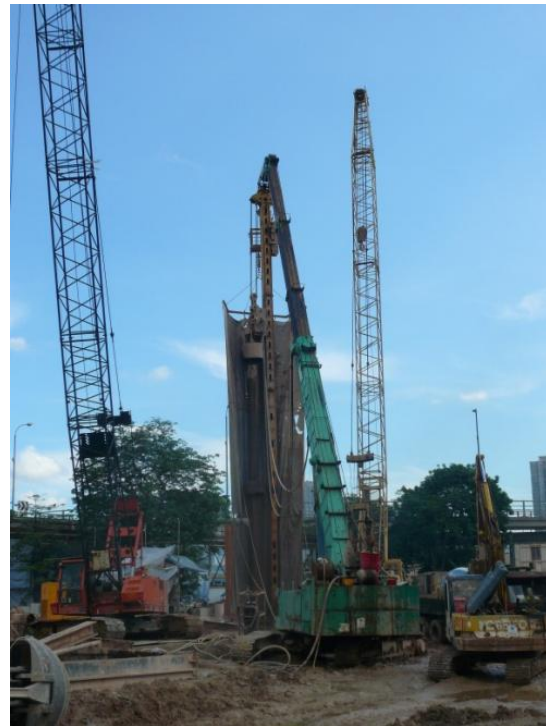
Figure 7. Pre-bored H-pile construction.
