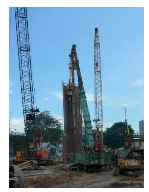
Figure 6. RCD mounted on casing top.
