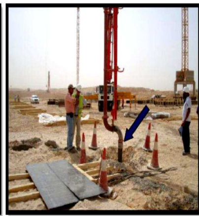
Figure 9.a. and b. Karst foundation bedrock treatments; cement grout injection, c. and d. high slump concrete filling.
