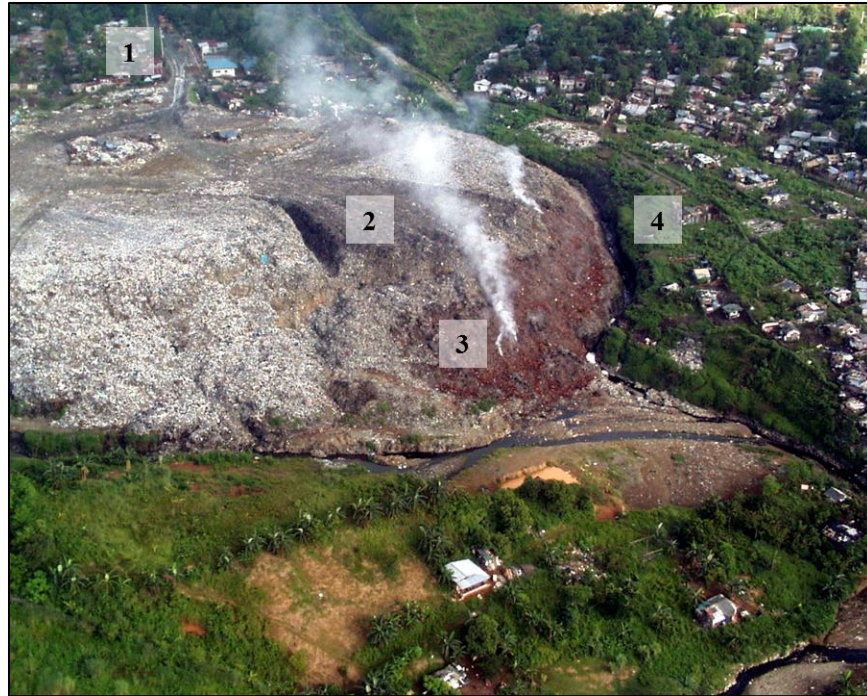
Figure 4. Stable landfill south of Payatas Landfill with waste slide showing smoke plumes (photo by S.M. Merry).
