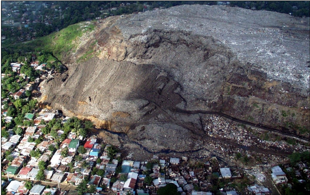
Figure 2. Aerial view of 12.7-hectare Payatas Landfill with slope failure and homes visible in foreground (photo by S.M. Merry).
