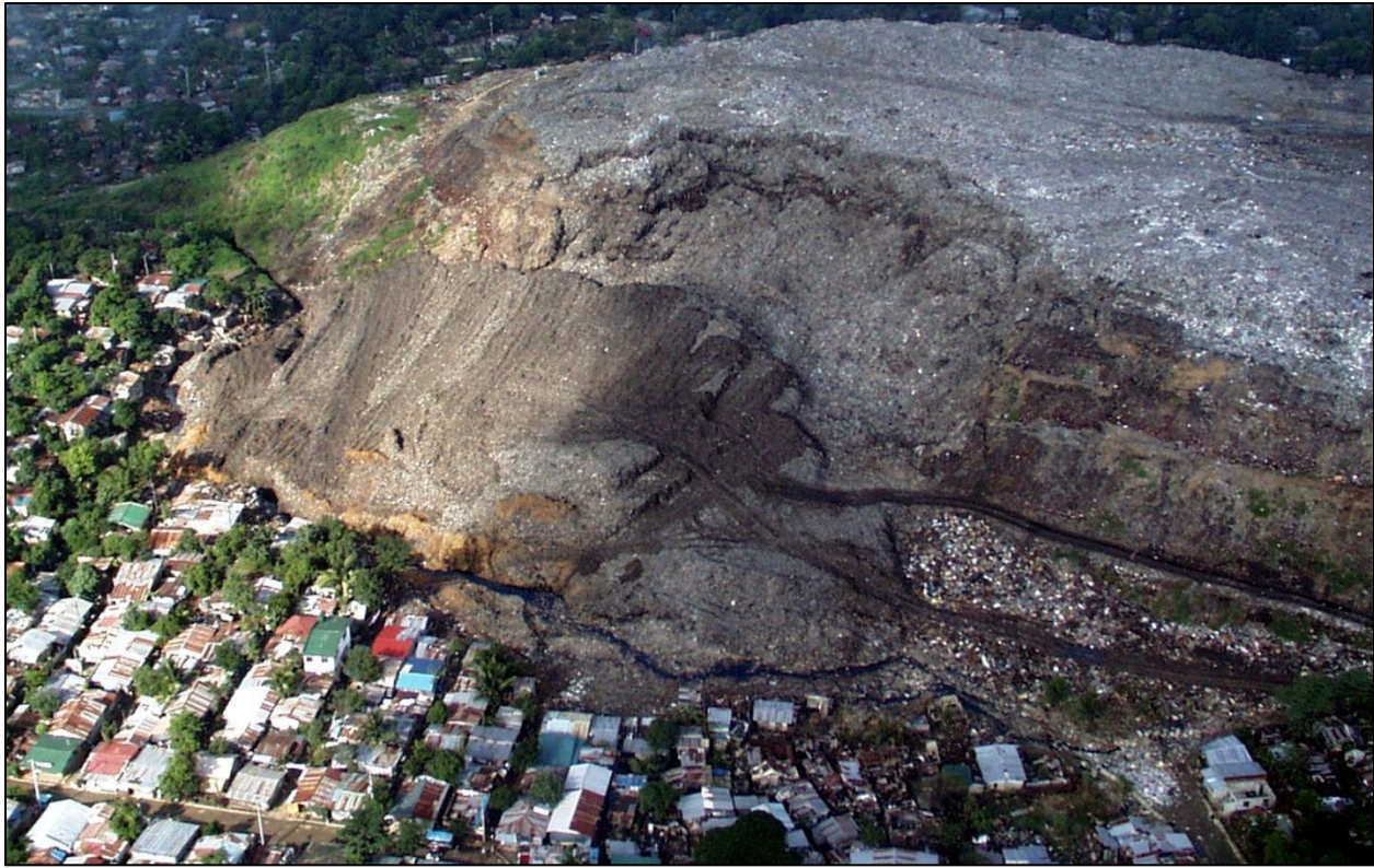
Figure 2. Aerial view of 12.7-hectare Payatas Landfill with slope failure and homes visible in foreground (photo by S.M. Merry).
