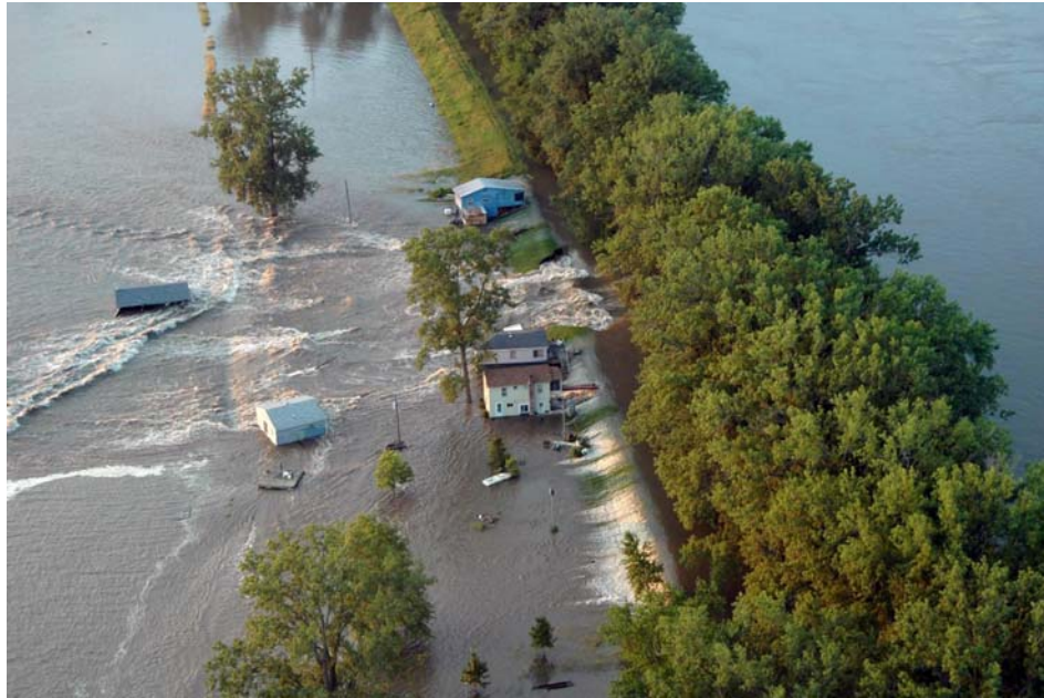
Figure 12. Winfield-Pin Oak breach (USACE St. Louis District 2008).
