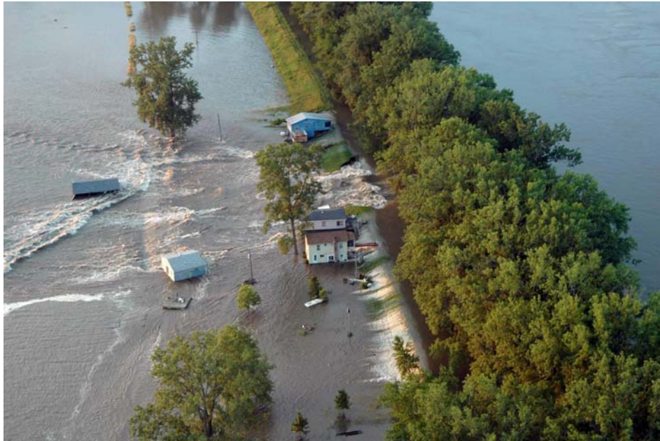
Figure 12. Winfield-Pin Oak breach (USACE St. Louis District 2008).
