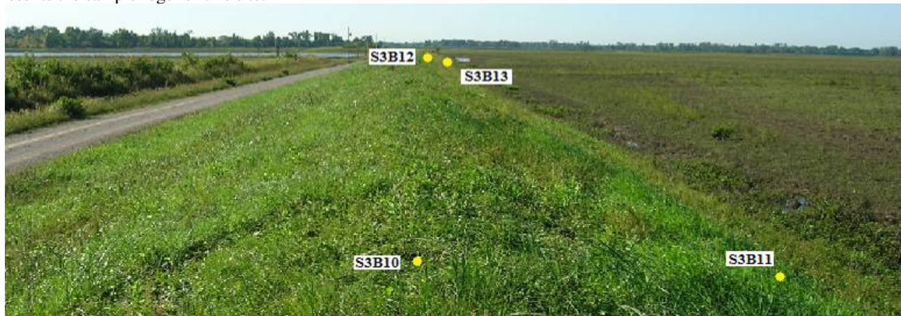
Figure 20. Brevator boring locations.
