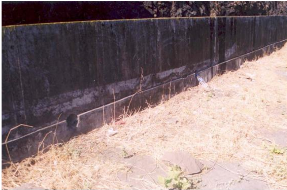
Figure 15. Drainage holes left open on embankment surface.
