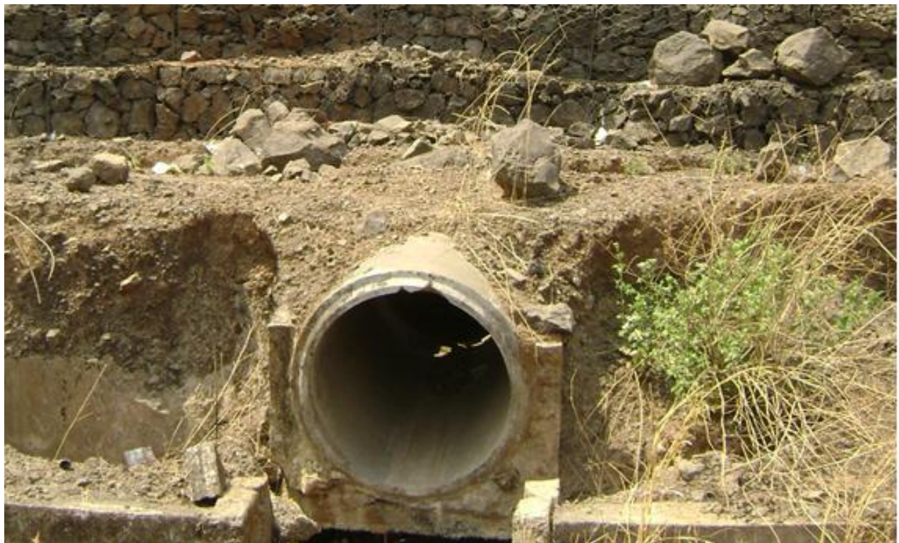
Figure 12. Pipe culvert without stepped chute.
