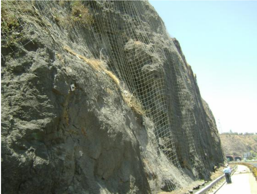
Figure 8. Remedial measures implemented on vertical slope (shotcrete and wire mesh).
