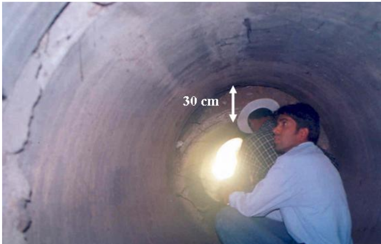
Figure 11. Dislodged pipe culvert.
