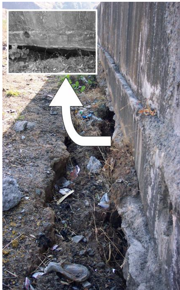
Figure 16. Embankment scoured below the crash barrier.
