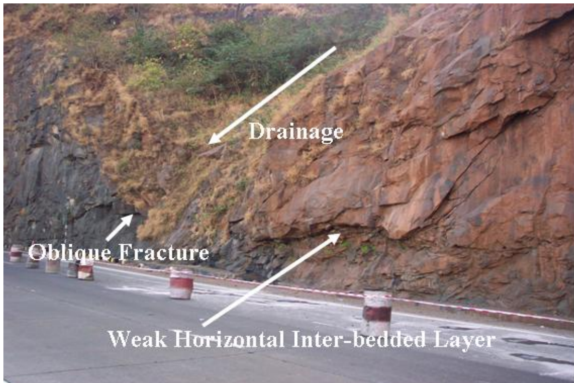
Figure 6. Intersection of oblique and sub-horizontal fractures.
