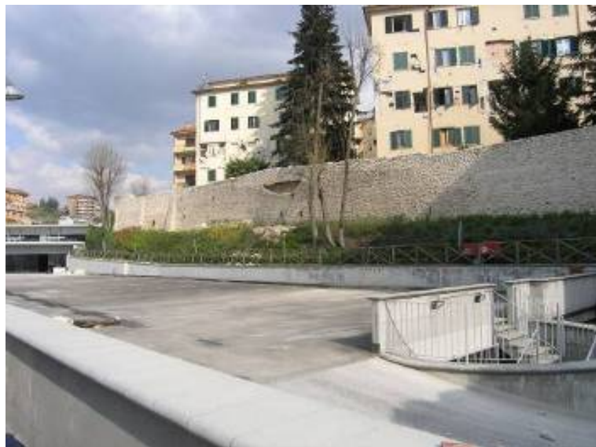
Figure 188. Damaged wall at downtown L'Aquila (42.356056°N, 13.389524°E).
