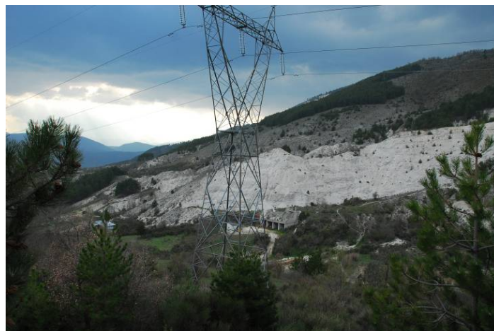
Figure 129. Quarry in Cataclasite with estimated 50^\circ slopes up to approximately 60 m high, located northeast of Colle (42.437N, 13.328E).
