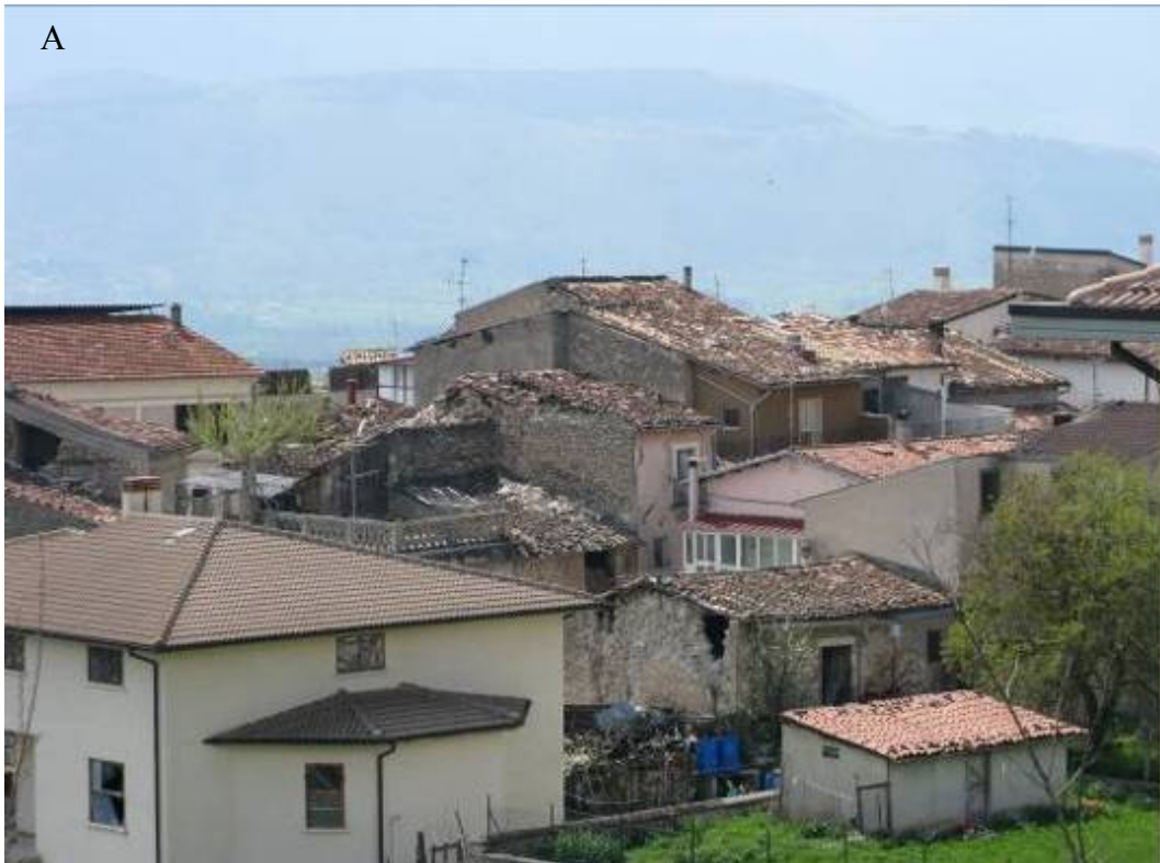
Figure 86. Poggio Picenze. (A) Variable damage (D3-D4) on masonry buildings of different style.
