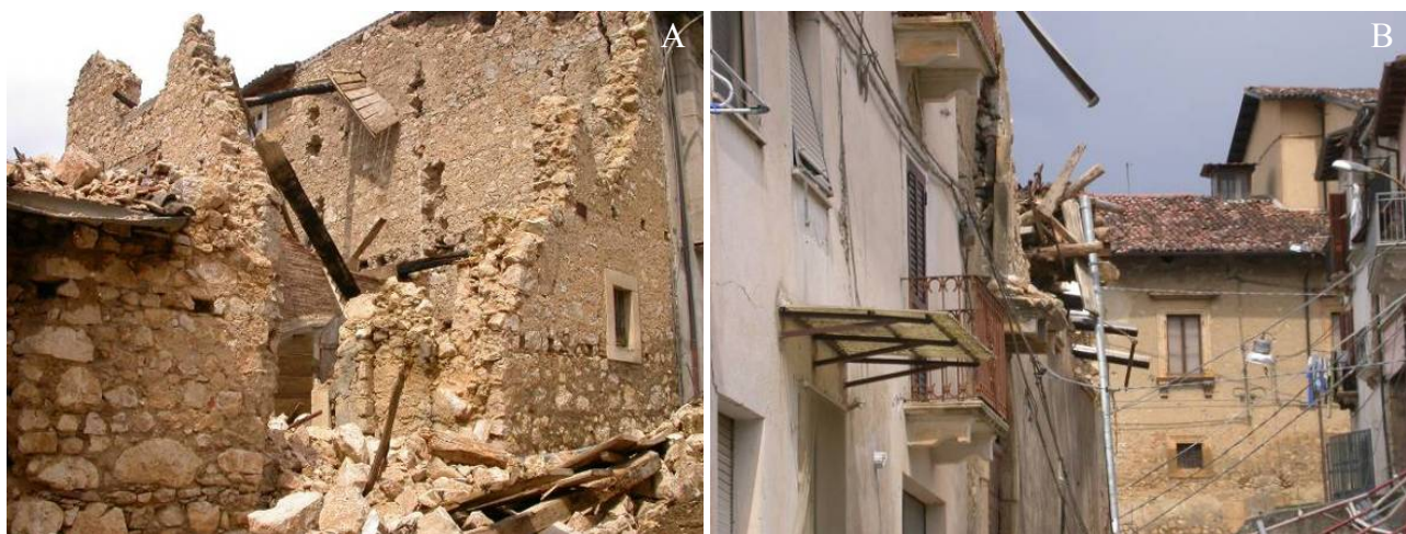
Figure 80. S. Eusanio Forconese. (A) Collapse of old masonry building (D5), (B) Partial collapse of masonry building (D4).
