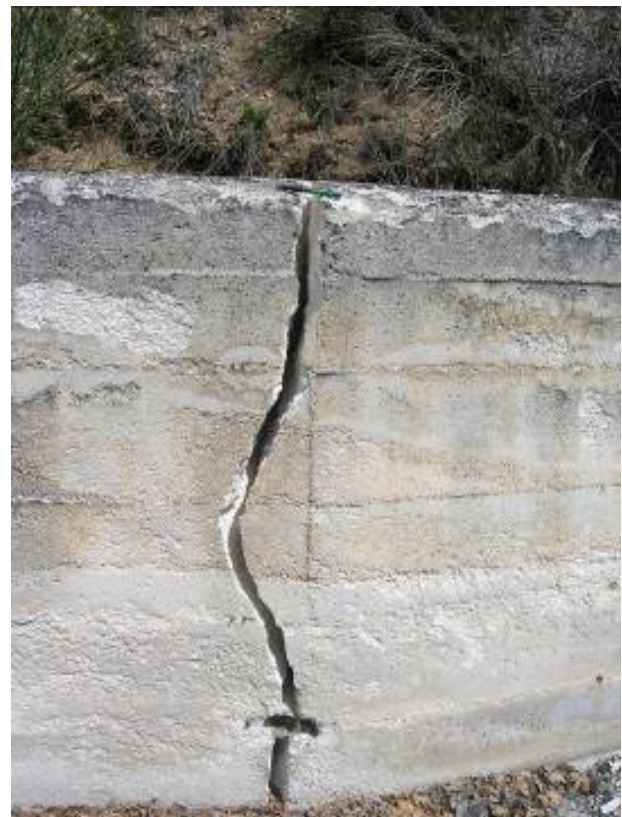
Figure 192. Ruptured retaining wall due to slope instability at SS80 highway between L'Aquila and Campotosto (42.418117°N, 13.351591°E).
