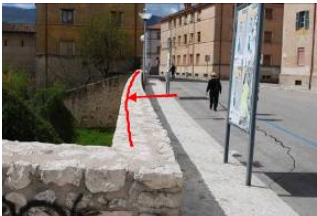
Figure 186. Stone masonry wall at L'Aquila city (42.348710°N, 13.403900°E). Note the (tolerable) outward movement at the center of the wall and the pavement cracks behind the wall.
