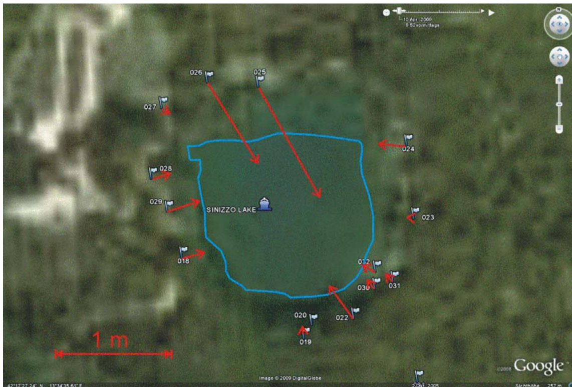
Figure 163. GPS waypoints indicating measurement locations around Lake Sinizzo. The red arrows indicate the orientation and maximum cumulative crack opening measured at each location.
