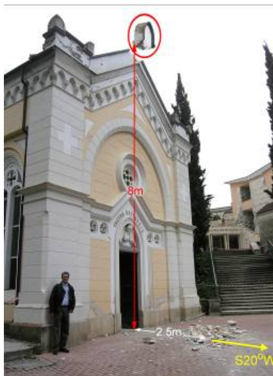
Figure 53. Fall of facade object at mortuary building.
