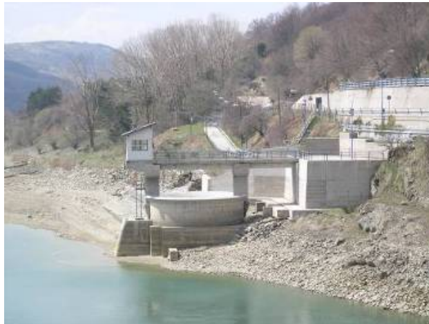
Figure 180. View of the outlet tower of Rio Fucino dam (42.535047°N, 13.410323°E).
