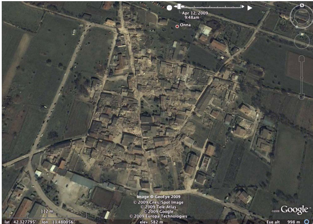
Figure 64. The village of Onna suffered D4–D5 damage in most of the unreinforced masonry structures. Reinforced concrete structures at the margins of the village performed well with only minor damage (D0-D2).
