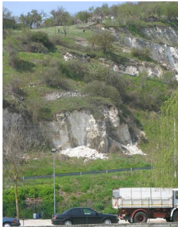
Figure 125. Slides on the eastern flank of the Bazzano hill (in the foreground SS17 highway) (42.34005N, 13.45560E).
