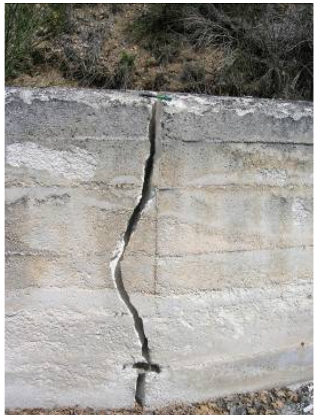
Figure 192. Ruptured retaining wall due to slope instability at SS80 highway between L'Aquila and Campotosto (42.418117°N, 13.351591°E).
