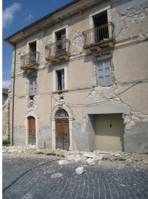
Figure 58. A typical heavily damaged structure in the lower elevation of Castelnuovo. Many structures in the lower elevation neighborhood had less observable damage. (42.2956°, 13.6274°).
