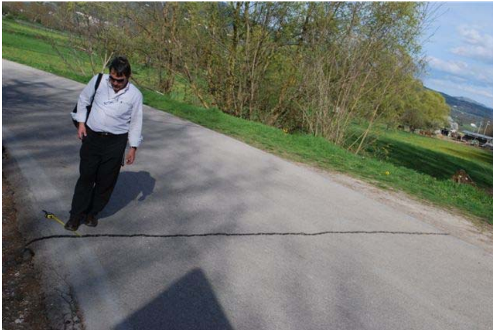
Figure 141. Characteristic crack developed in bridge approach road directly south of Onna, at distances of 15 m to 160 m from the Aterno River (42.324N, 13.478E).
