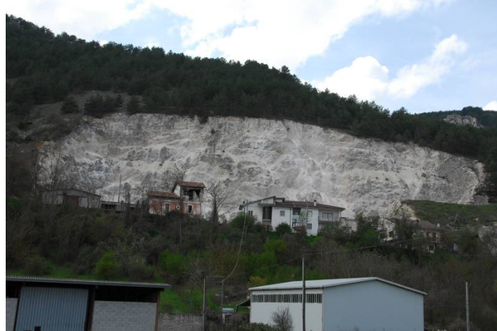
Figure 127. Quarry in Cataclasite with estimated 60^\circ slopes up to approximately 35 m high, located in Fossa (42.300N, 13.485E).
