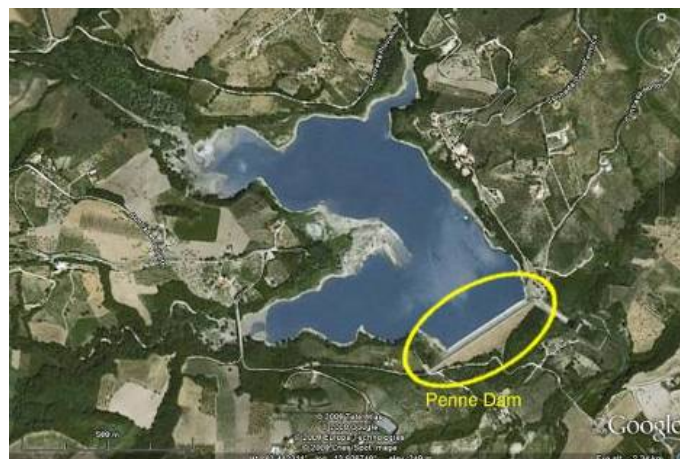
Figure 184. Location map for Penne reservoir and dam (42.438809°N, 13.913265°E).
