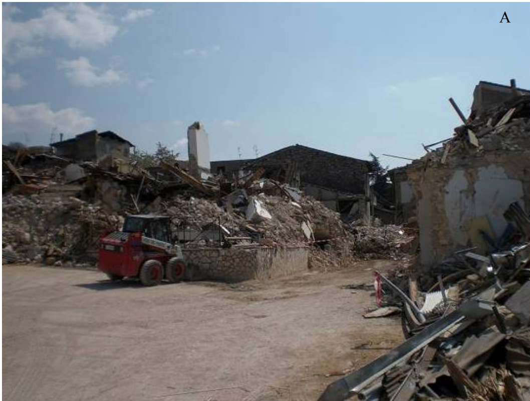
Figure 72. San Gregorio. (A) View of the historic center with collapsed masonry buildings.
