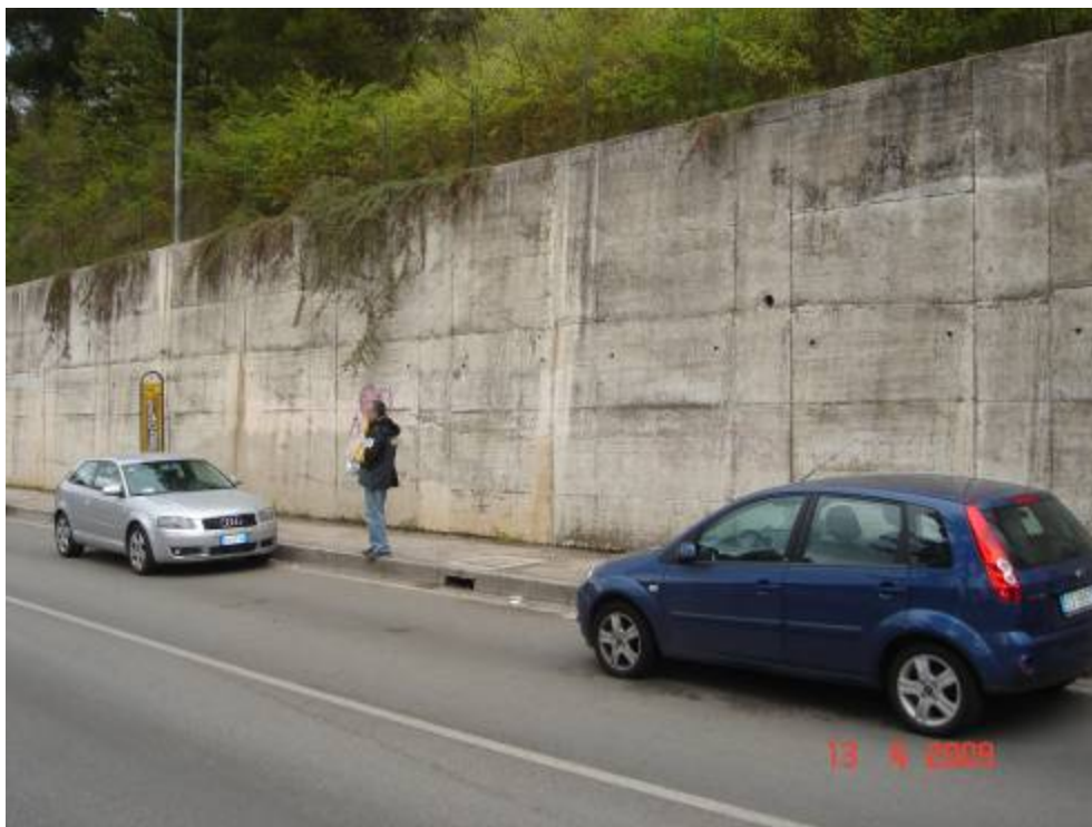
Figure 194. Undamaged retaining wall at the city of L'Aquila (42.343672°N, 13.398821°E).
