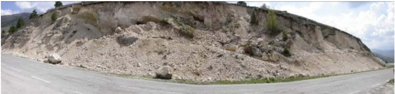
Figure 124. Slides and topples along the road from Barisciano to S.Stefano.(DC-11-1; 42.3349N, 13.5796E).
