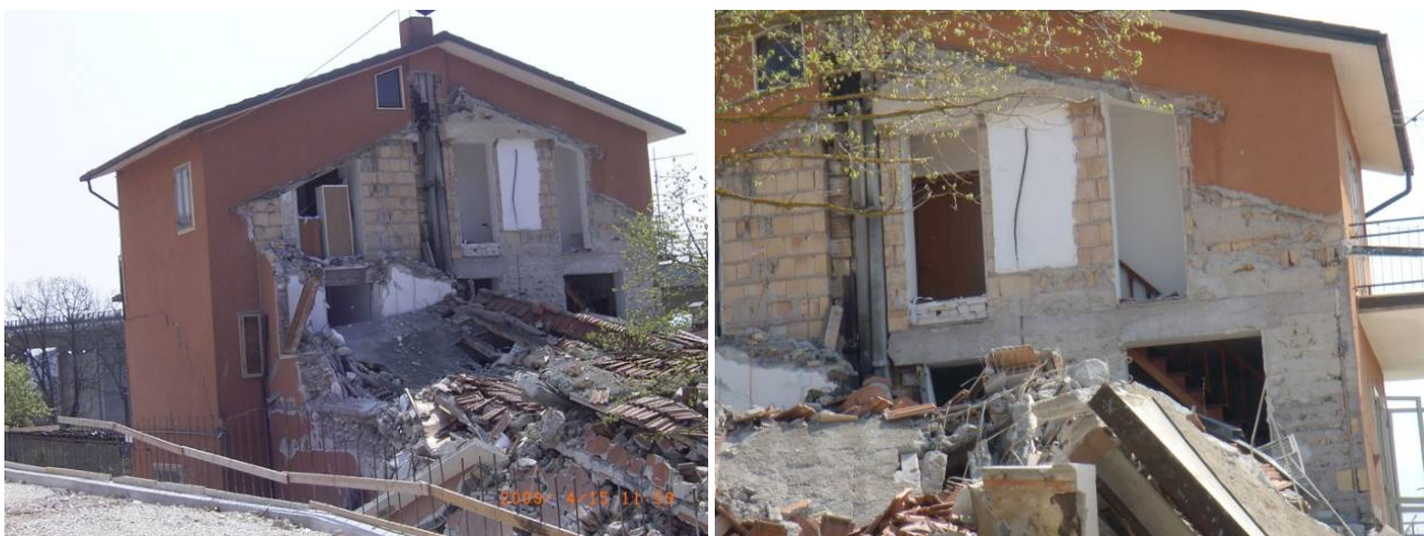
Figure 104. Masonry structure at waypoint GB-82-1.
