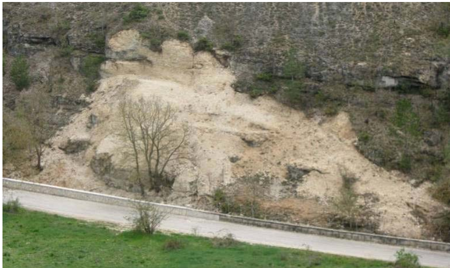
Figure 122. Ravelling along the road from S. Demetrio to Lake Sinizzo (42.28845N,13.56442E).
