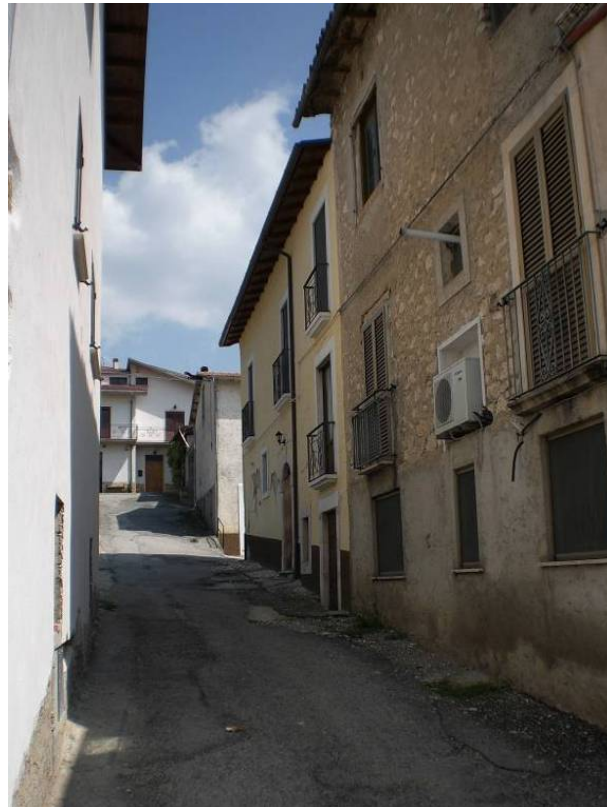
Figure 73. San Gregorio western part: masonry buildings with minor damages.
