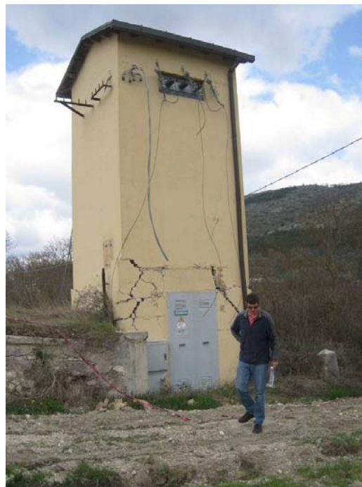
Figure 57. Heavily damaged seismometer station box (not in use at the time of the earthquake, no recording) on the northeast valley beneath the town of Castelnovo. ( 42.2982^{\circ} , 13.6295^{\circ} ).
