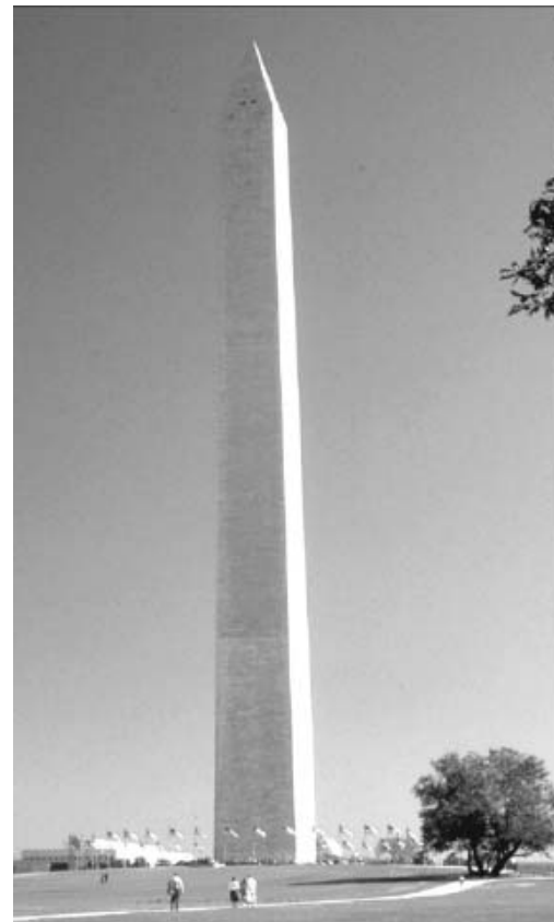
Figure 2b. Final design – constructed monument.
