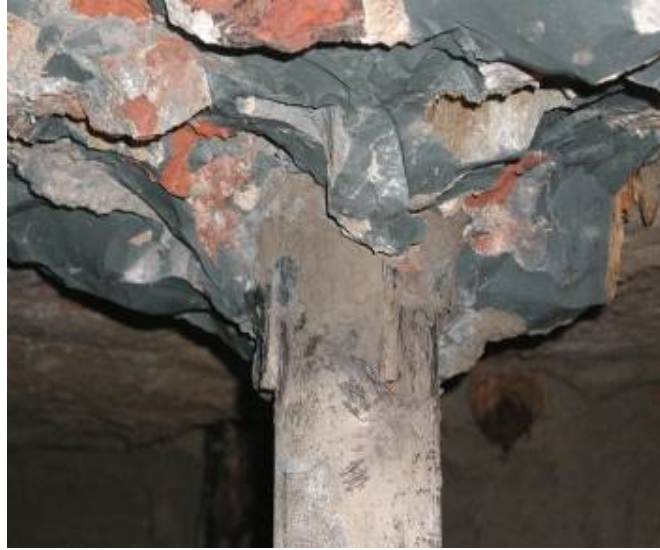
Figure 18. Bored pile with tube reinforcement viewed from underneath foundation.
