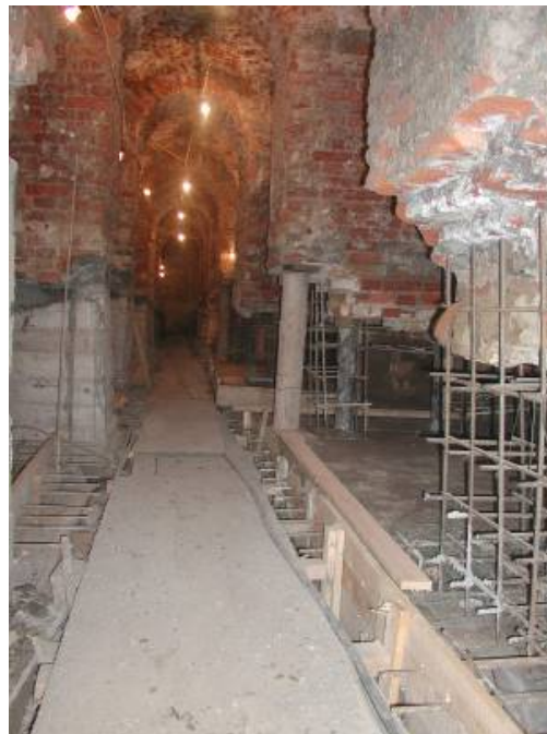
Figure 17. Deepening of the basements by 1.0-1.5 m.
