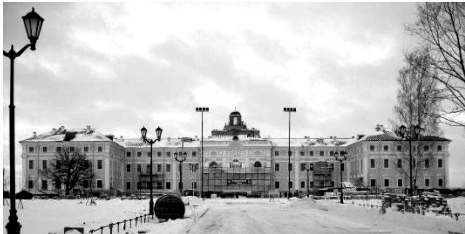
Figure 19. Konstantinovsky Palace, south façade. View of a final reconstruction stage (January 2003).
