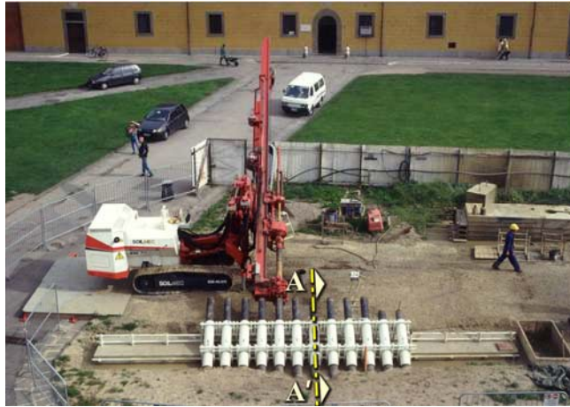
Figure 9. Holes for preliminary underexcavation.
