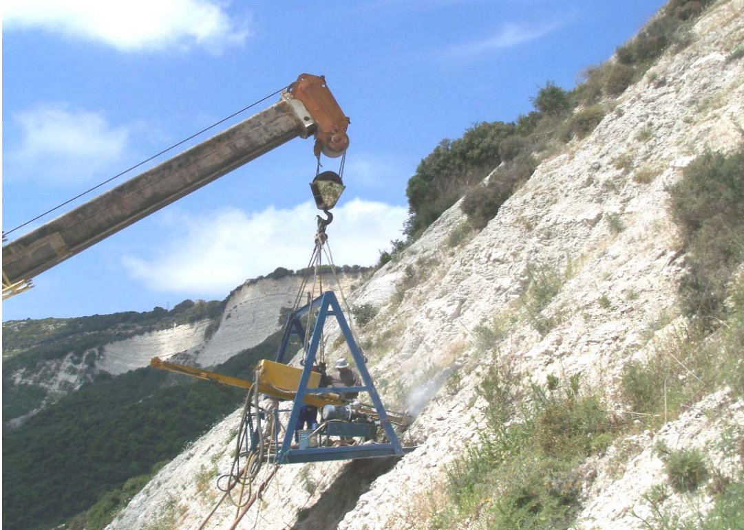
Figure- 13. Installation of the Nails/bolts Along the Western Slopes.
