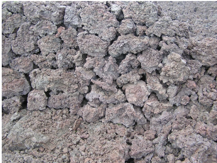
Figure 40. Location 11, Saddle Road (Hwy 200). Stacked rock wall of a 'a clinker.
