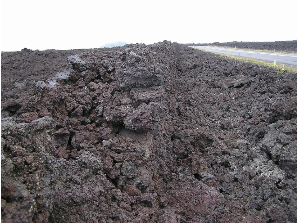
Figure 9. Location 11, Saddle Road (Hwy 200). Lava flow of a'a clinker and dry stacked wall of clinker composed of a'a blocks.
