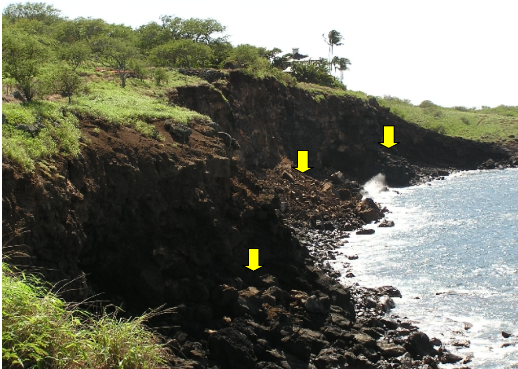
Figure 34. Location 23, failed cliffs (arrowed) south of Honoipu Landing (Ala Kuakini Trail).
