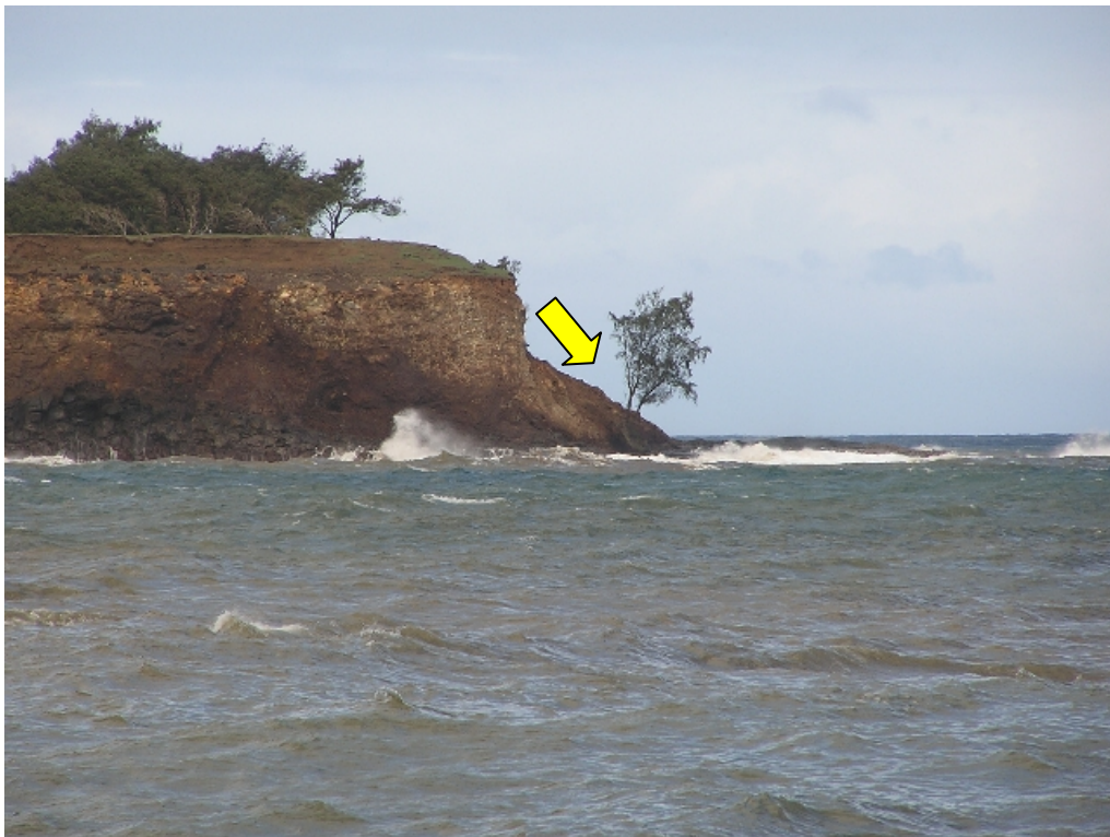
Figure 33. Headland to the northwest of Location 19, Kēōkea Bay. Cliff top slid into the ocean, indicated by the displaced tree and the mostly submerged toe debris.
