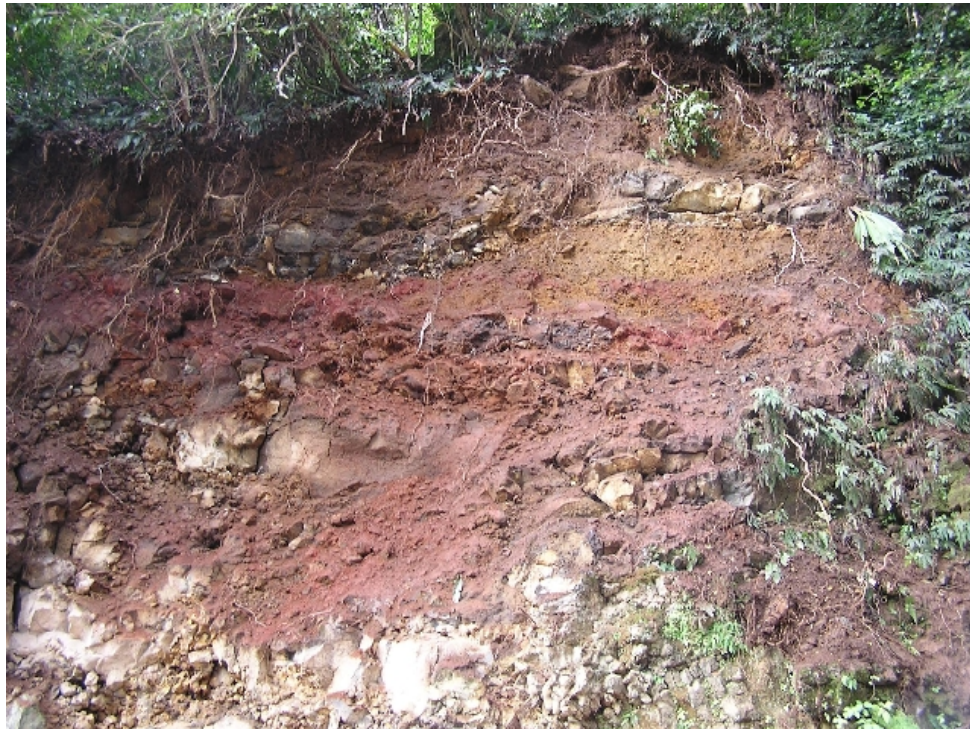
Figure 26. Location 4: old Hwy 11 near Ōōkala. Failure of soil above rock. Note inclusions of corestone rocks within soil.
