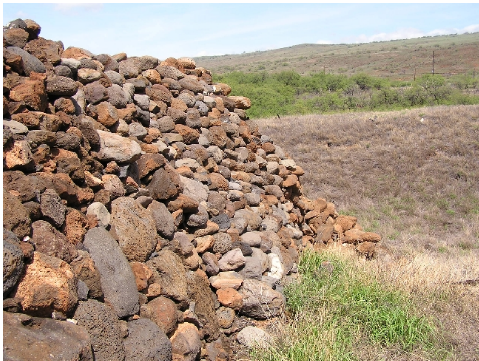
Figure 52. Location 29, NE corner Mailekini heiau. In foreground: typical intact face inclined at about 50 degrees. In background, toe of raveled face shown in Figure 56.
