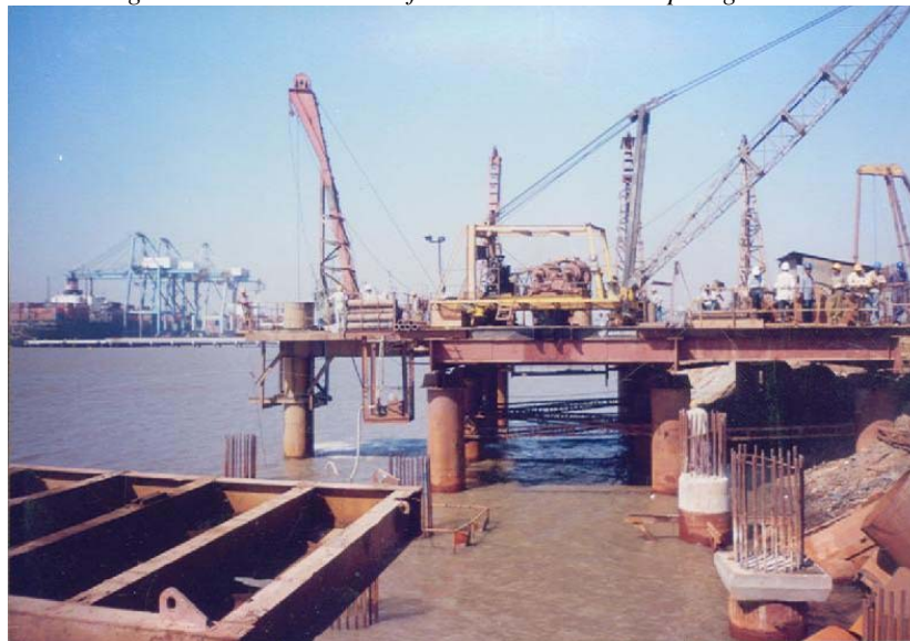
Figure 11. Construction of Piles.
