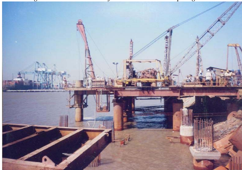
Figure 11. Construction of Piles.
