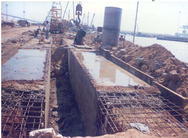
Figure 10. Construction Of Guide Walls For Diaphragm Wall.
