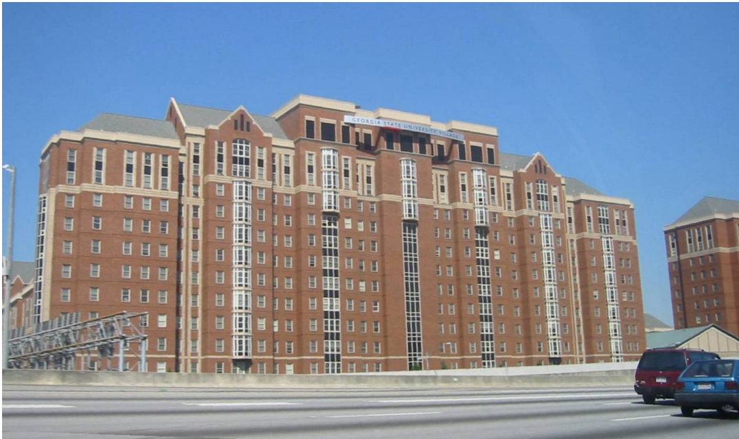
Figure 11. View of Dorm B looking west from combined interstates I-75/I-85.
