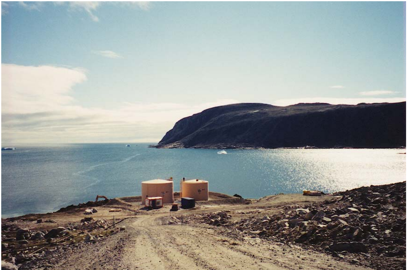
Figure 2. View looking toward ocean showing existing fuel tanks.
