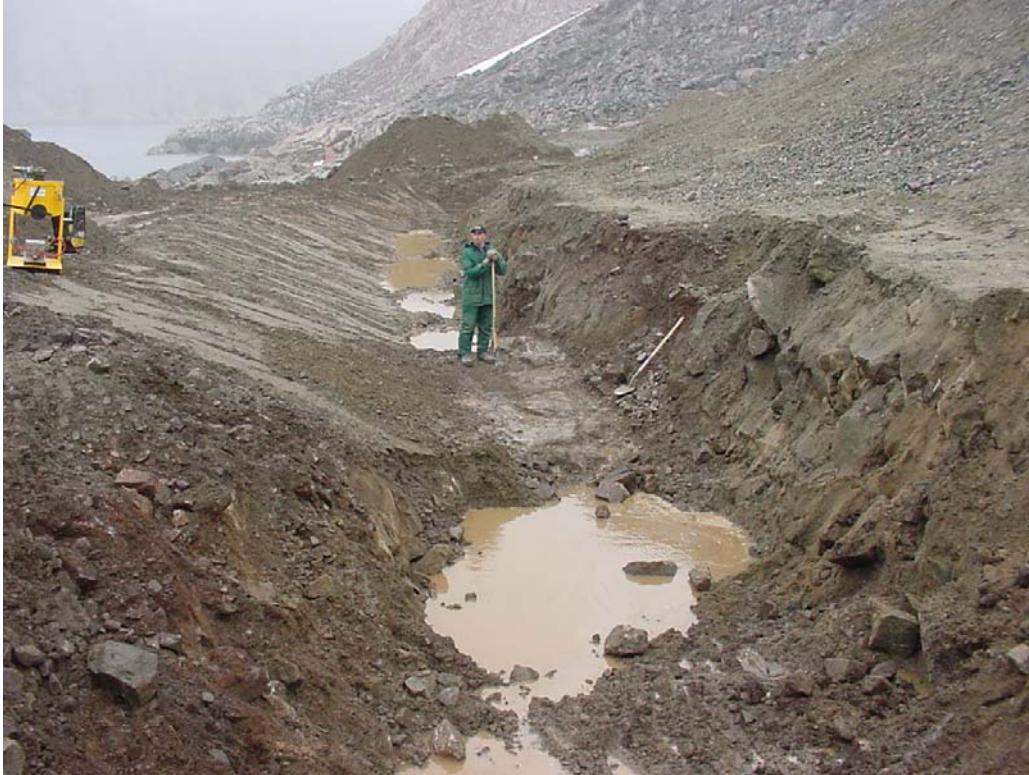
Figure 5. Photograph of trench excavation illustrating bedrock encountered at trench bottom.
