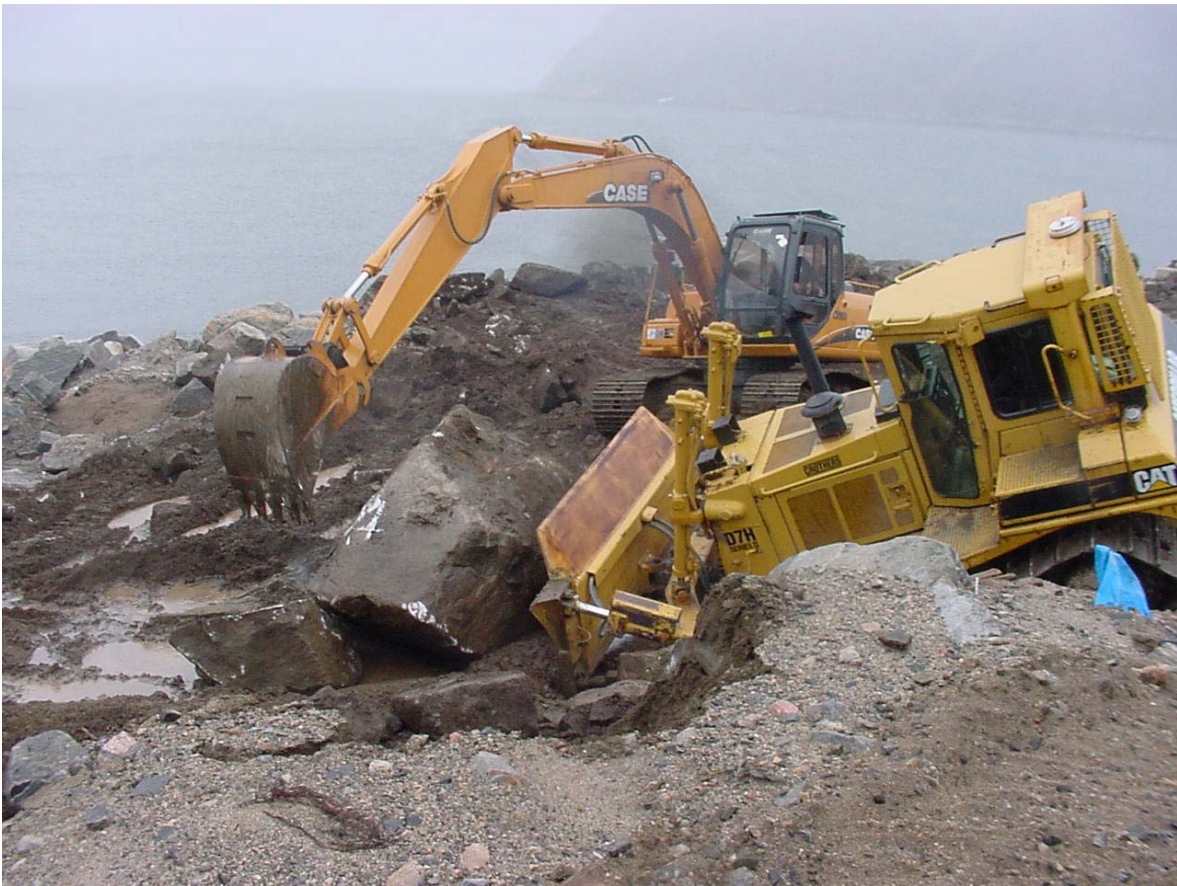
Figure 4. Photograph illustrating large boulders encountered at east end of trench excavation.
