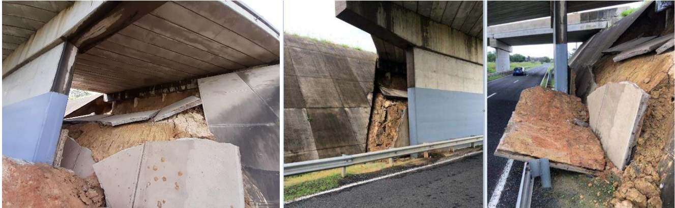
Figure 2. Abutment condition after failure.
