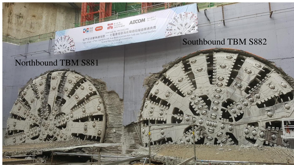
Figure 9. 14 m diameter slurry mix-shield TBMs.
